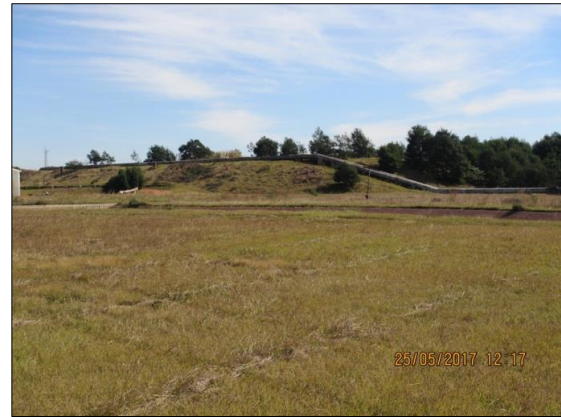
Figure 11: View of High-level Water Return Dam servitude, showing pipeline and ditch
