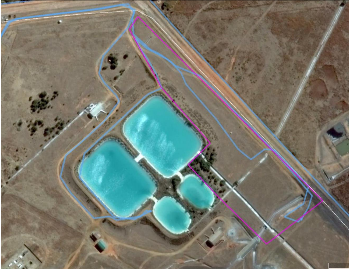
Figure 21: Tracklog for High-level Water Return dam servitude
