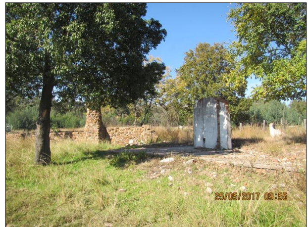
Figure 23: DUV001, showing boundary wall and remains of structure outside the wall
