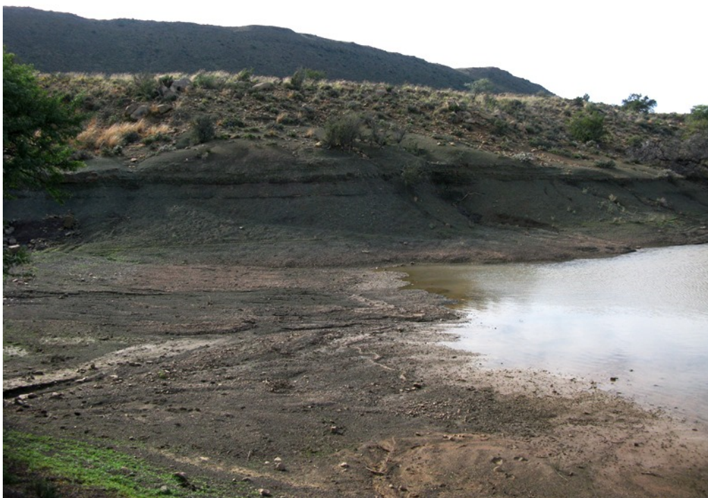
Figure 2: View north-eastwards across the existing MR599/41.0/0.02R (Almond 2015: 4)
