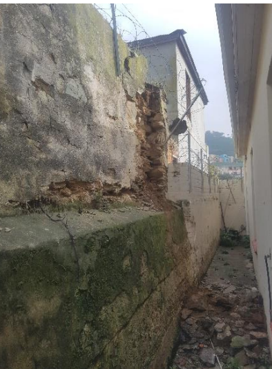
Side space west looking north
