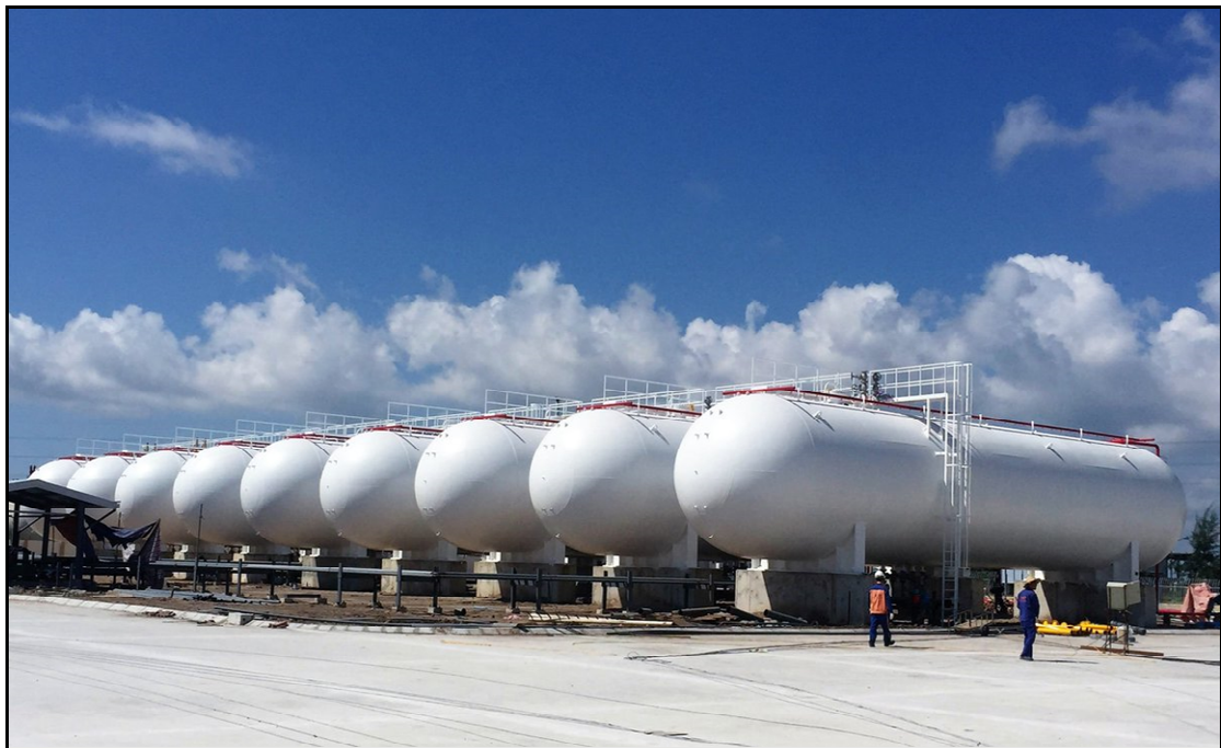
Figure 6: Example of storage tanks at a LPG depot. Photo: Engineering News.
