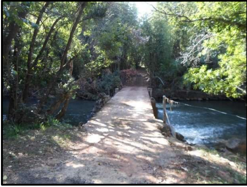
Figure 8.8. Bridge at SCH028
