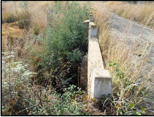
Figure 8.2. General site conditions at SCH 005.
