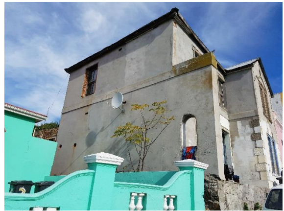
North east facade
