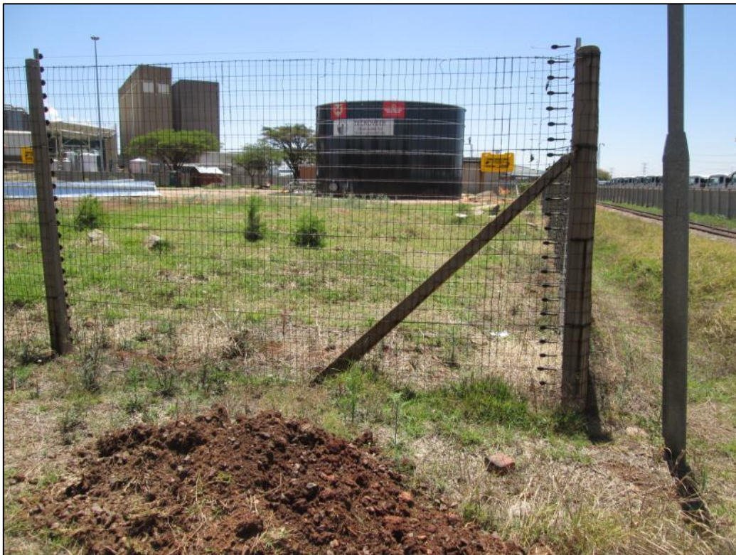
Figure 7 – View of the pipeline route outside of the concrete wall, but still within the fenced-off area of SAB. The pipeline will run just on the inside of the fence, next to the fence line and will cross the fence at this point
