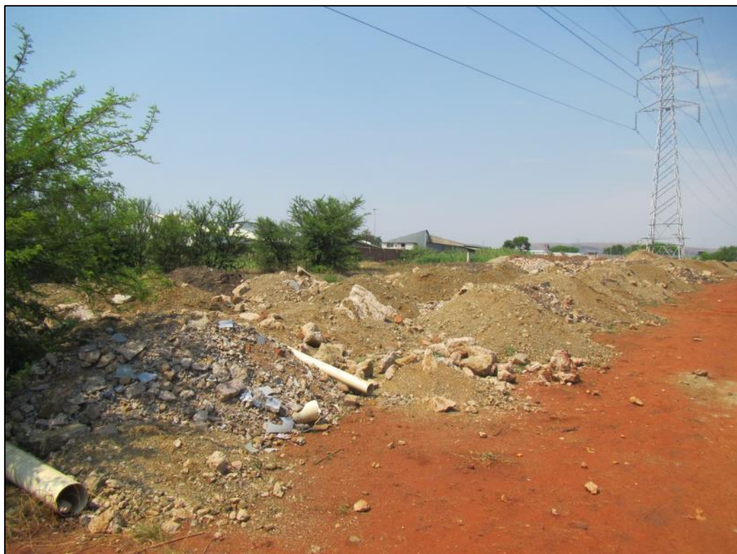
Figure 15 – View of the mid-section of the pipeline route showing the recent dumping of soil and rubble as well as the overhead powerline running along the route.
