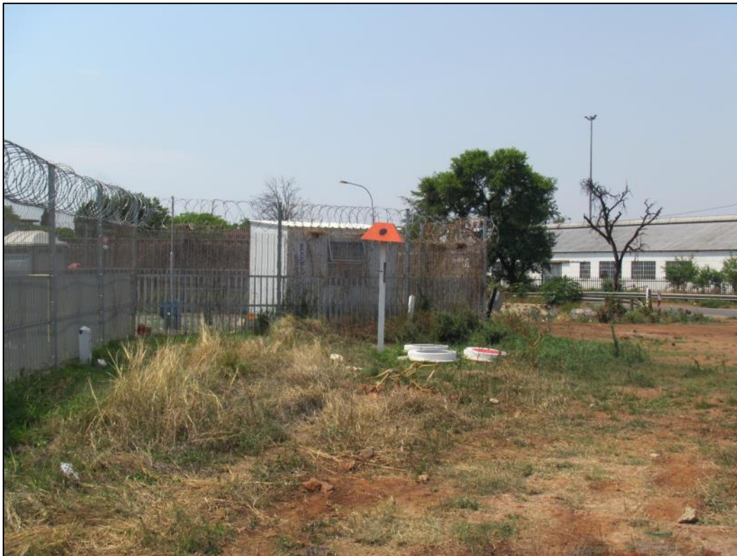
Figure 18 – View of the end-point of the pipeline route, where it will tie in to the existing Sasol PRS
