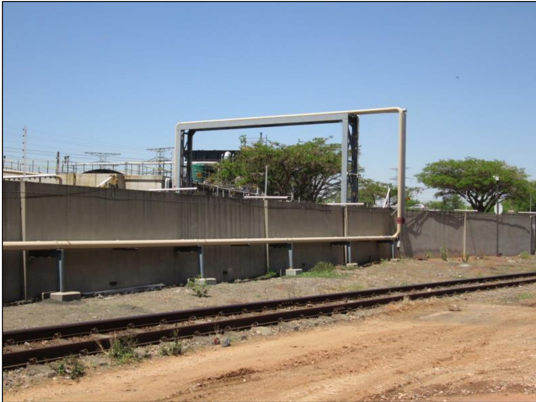
Figure 6 – View of the existing pipeline and pipeline bridge across the concrete wall. The new pipeline will cross the wall at the same spot.
