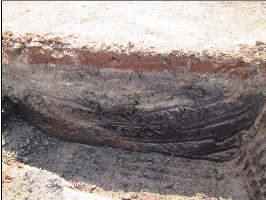
Figure 16- View of another test pit located in the middle of the southern section, which indicates the disturbed nature of the subsoil
