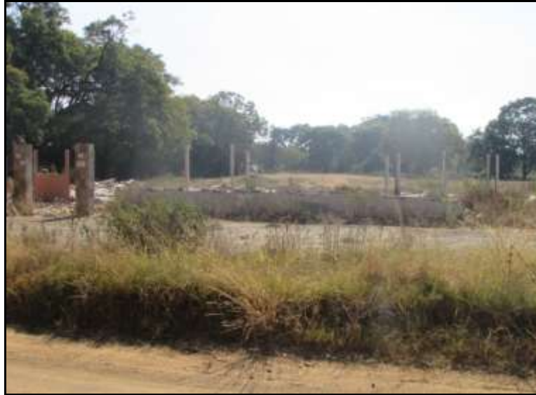
Fig.19: The foundations of another recent structure.
