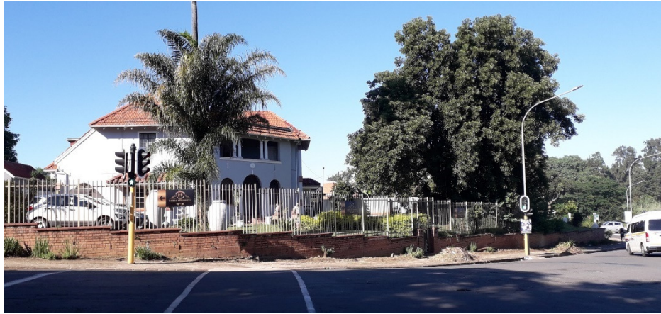
Fig. 4. View across New England Rd
