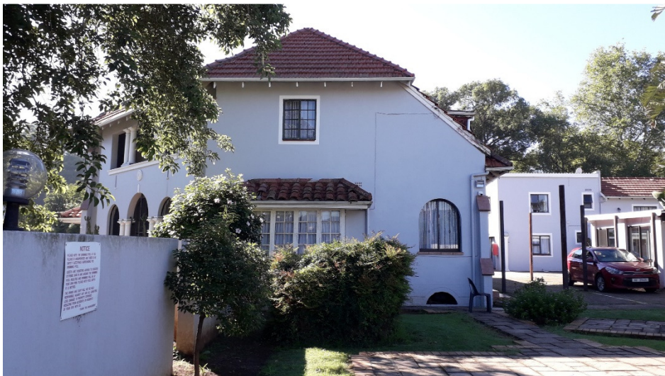
Fig. 12. Existing building – elevation facing the pool, development site to the right
