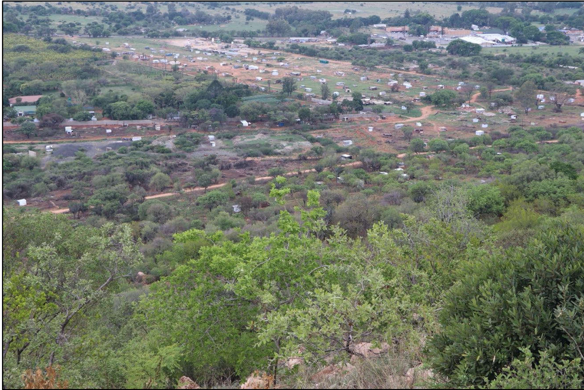
Figure 4 – General view into the north-east showing the more level areas of the study area. The small corrugated iron structures and cleared stands from the informal occupation of the property can be seen. In the background, near the top centre of the photograph, the brickfield that is located on the far north-eastern end of the study area is visible.
