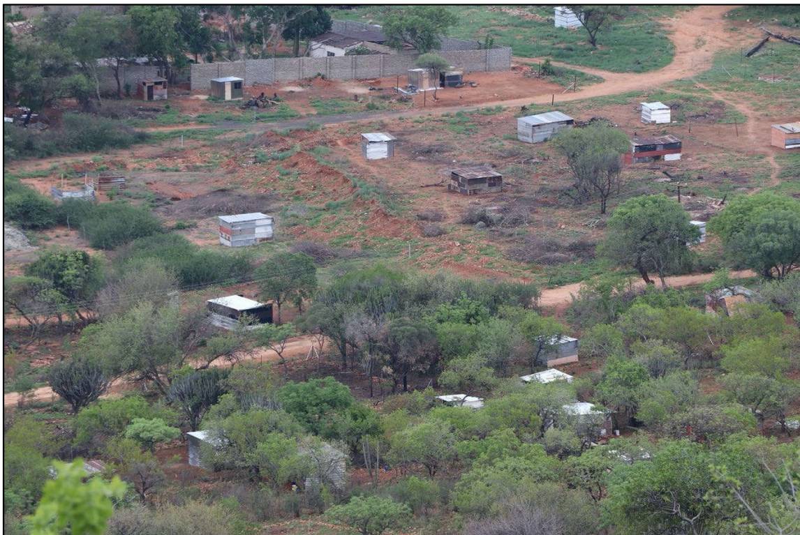
Figure 5 – Closer view of a section of the level areas from within the study area. The cleared stands and associated corrugated iron structures can be seen. This photograph was also taken in a north-eastern direction.
