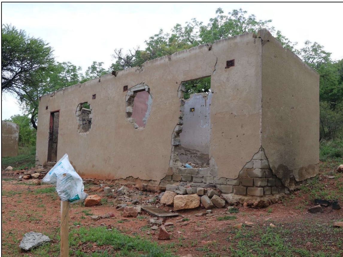
Figure 41 – Closer view of one of the structures from site BSCH 11.
