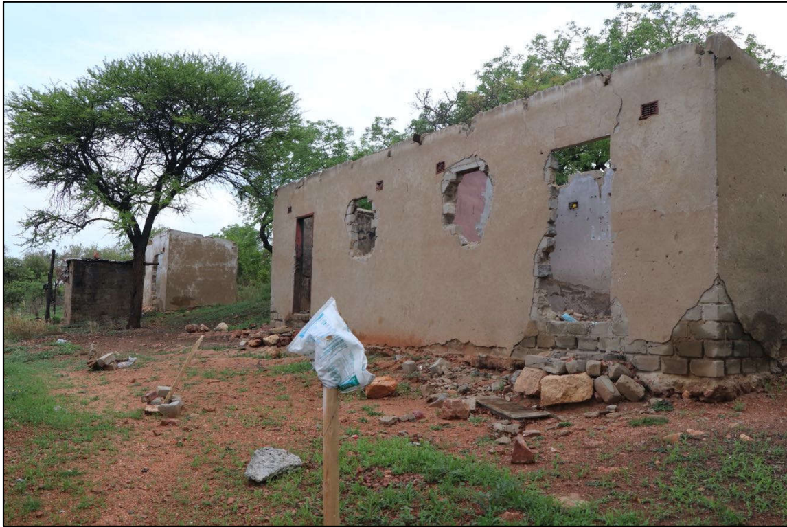
Figure 40 - General view of two of the structures from site BSCH 11.
