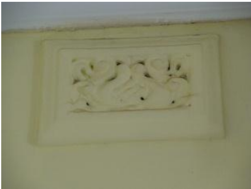
Figure 16: One of the moulded, decorative, airvents.
