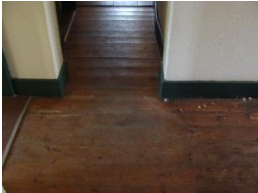
Figure 34: Original wood flooring in some sections.
