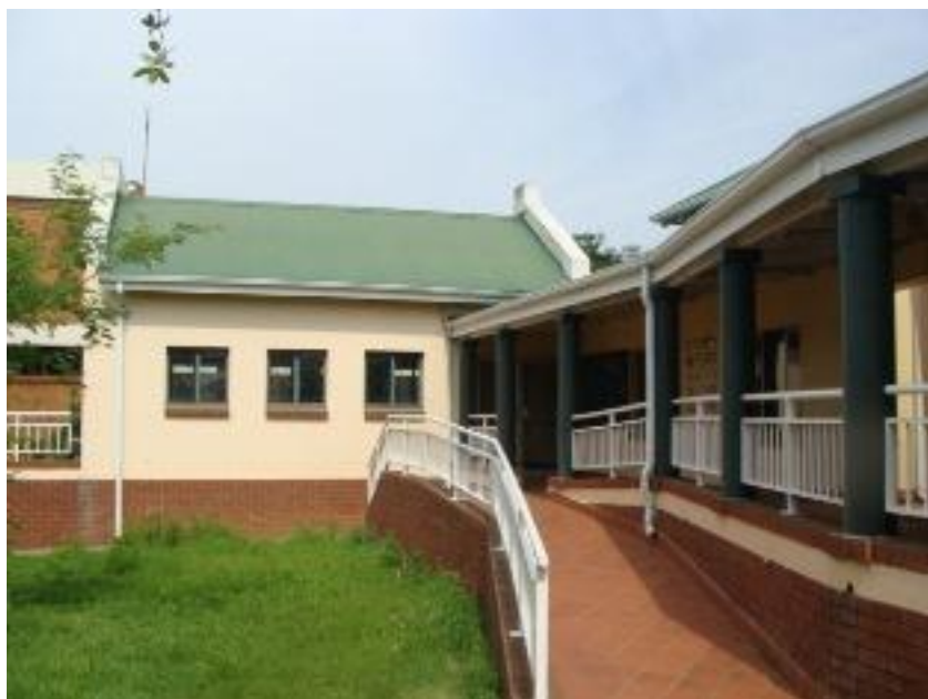
Figure 24: Closer-view of new additions (class/lecture rooms).
