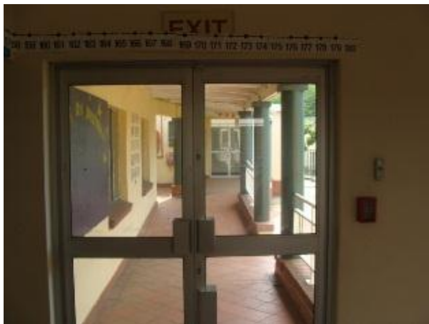
Figure 32: View of class room and stoep.
