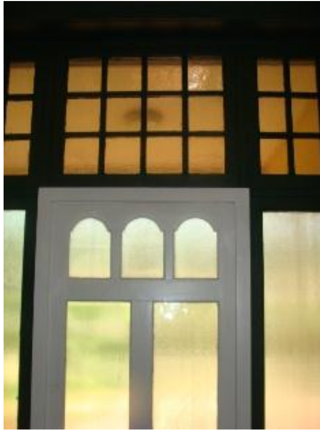
Figure 33: View of front door and glass panels.
