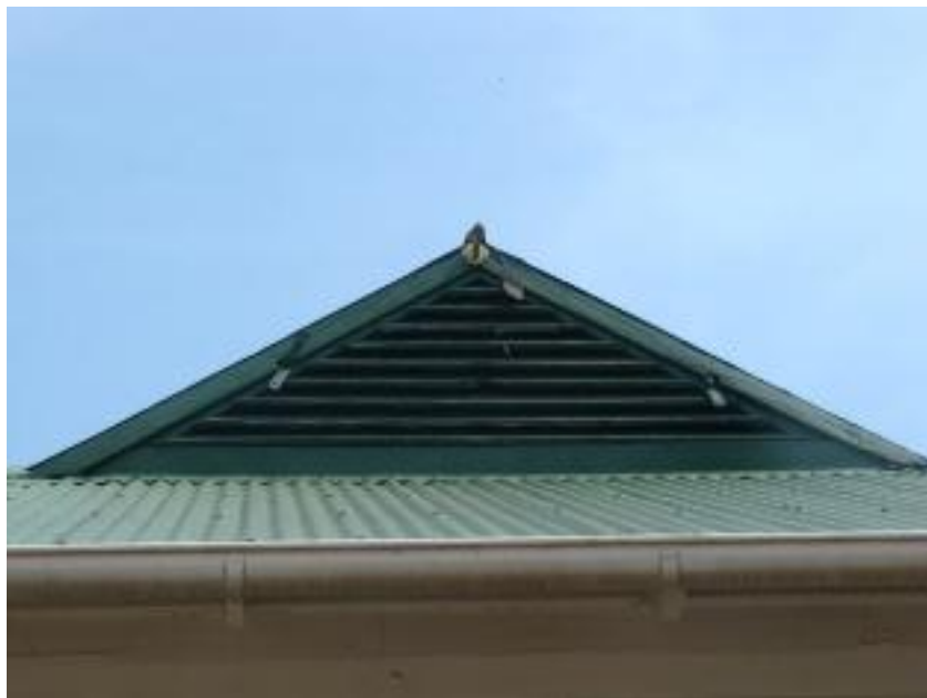
Figure 12: View of section of original roof.
