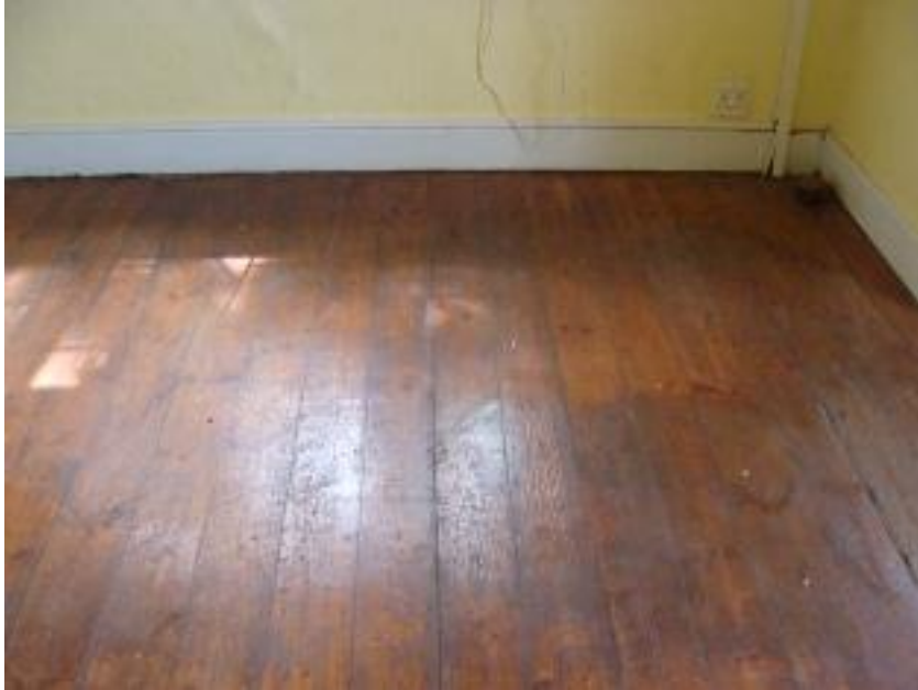
Figure 15: Original wood flooring in some sections.
