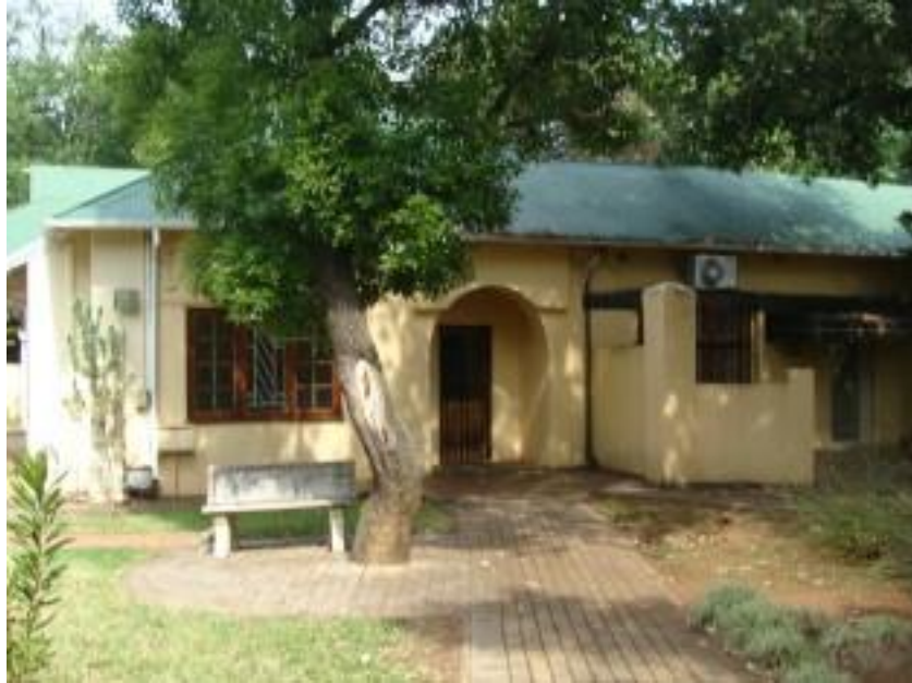
Figure 11: View of eastern side of the house.
