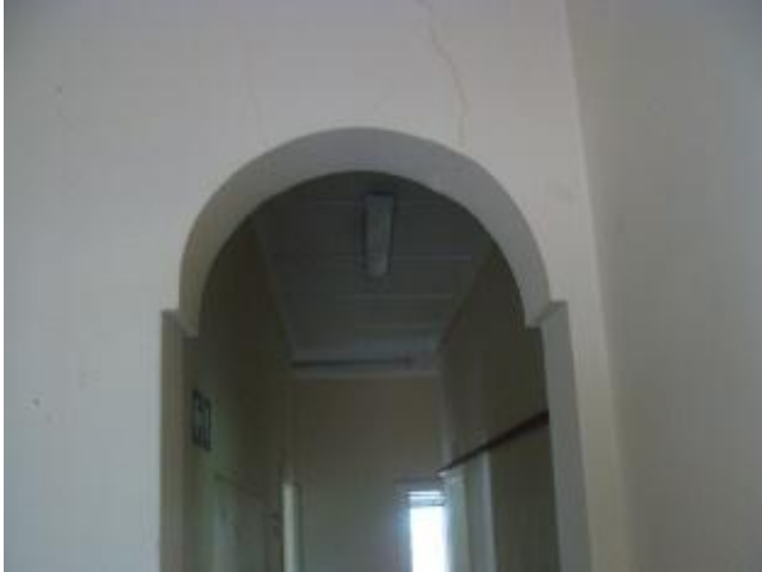
Figure 17: One of the original door arches.
