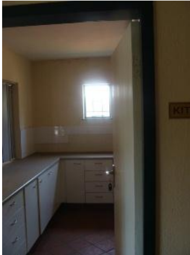
Figure 31: Kitchen area in American School.
