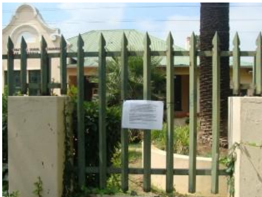
Figure 41: Site Notice in front of American School erf.
