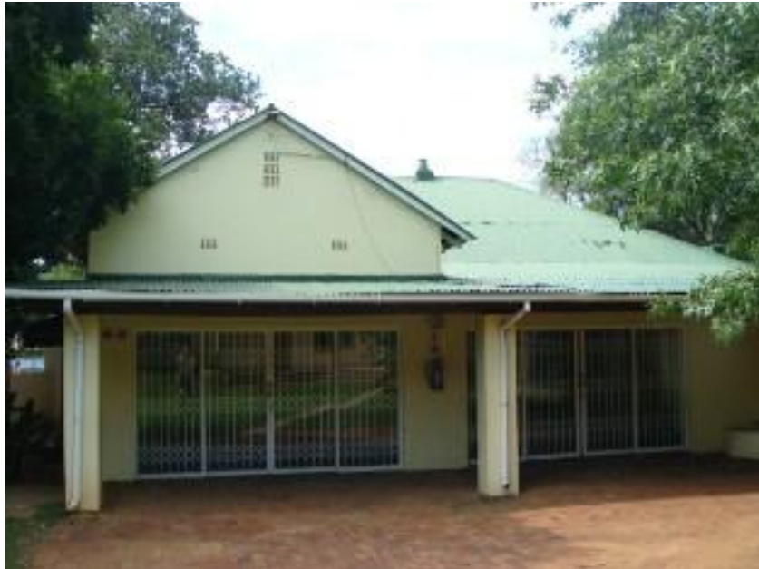
Figure 13: View from back of house. This section has been recently added.
