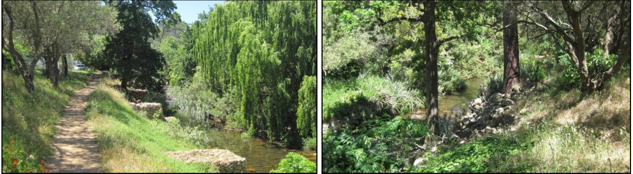
Intervention site 300-001 gabions (existing can be seen at left), Intervention site 300-002 tree roots
