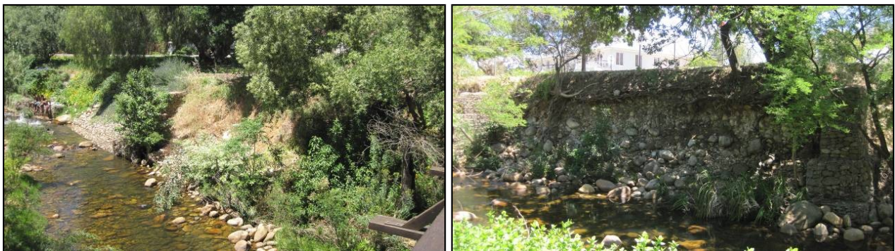
Intervention site 300-005 with existing gabions, Intervention site 300-006 with existing gabions
