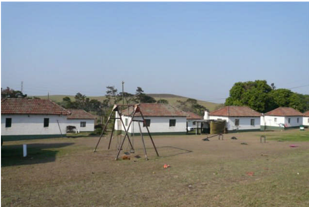
Plate 2. Inyaninga Barracks (South).
