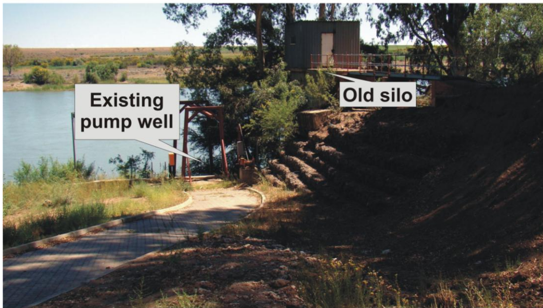
Figure 4. Existing infrastructure at the water abstraction facility.
