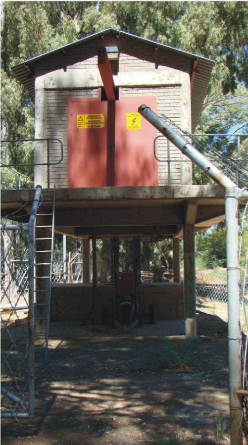
Figure 5. The pump house, looking east (above) and south (below, left).
