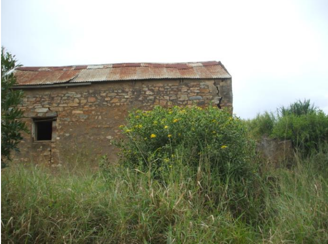
Figure 18b: Church building alongside road; near Varnam Elevation: 1421 ft S 33° 19' 33.8" E 26° 38' 17.4"
