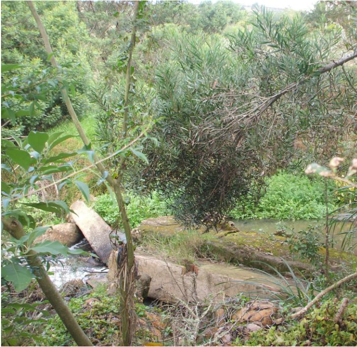
Figure 22b: broken weir on Willow Glen Annexe
