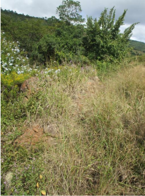
Figure 18a: Remains of school building alongside road; only foundations visible and some bricks and stones Elevation: 1513ft S 33° 19' 21" E 26° 36' 11"
