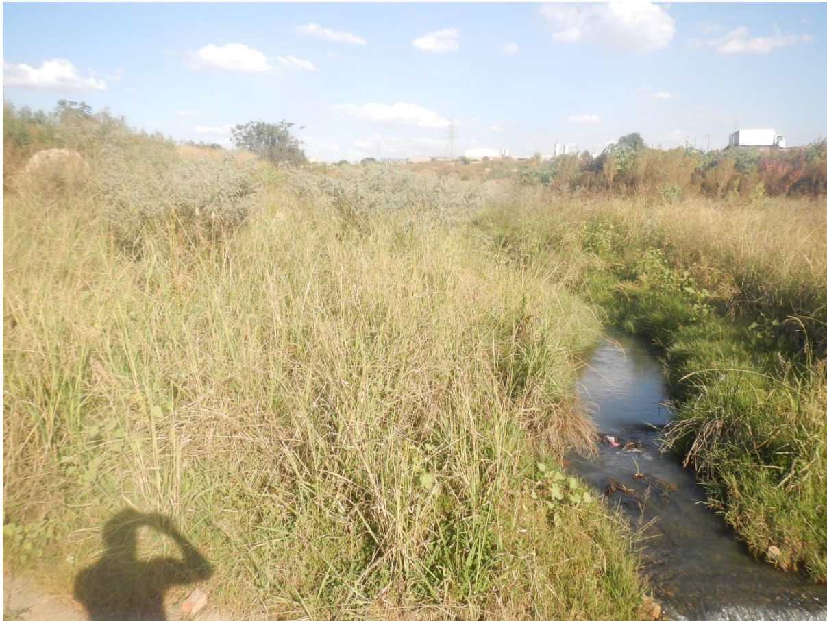
Figure 10 : A view of part of the pipeline route
