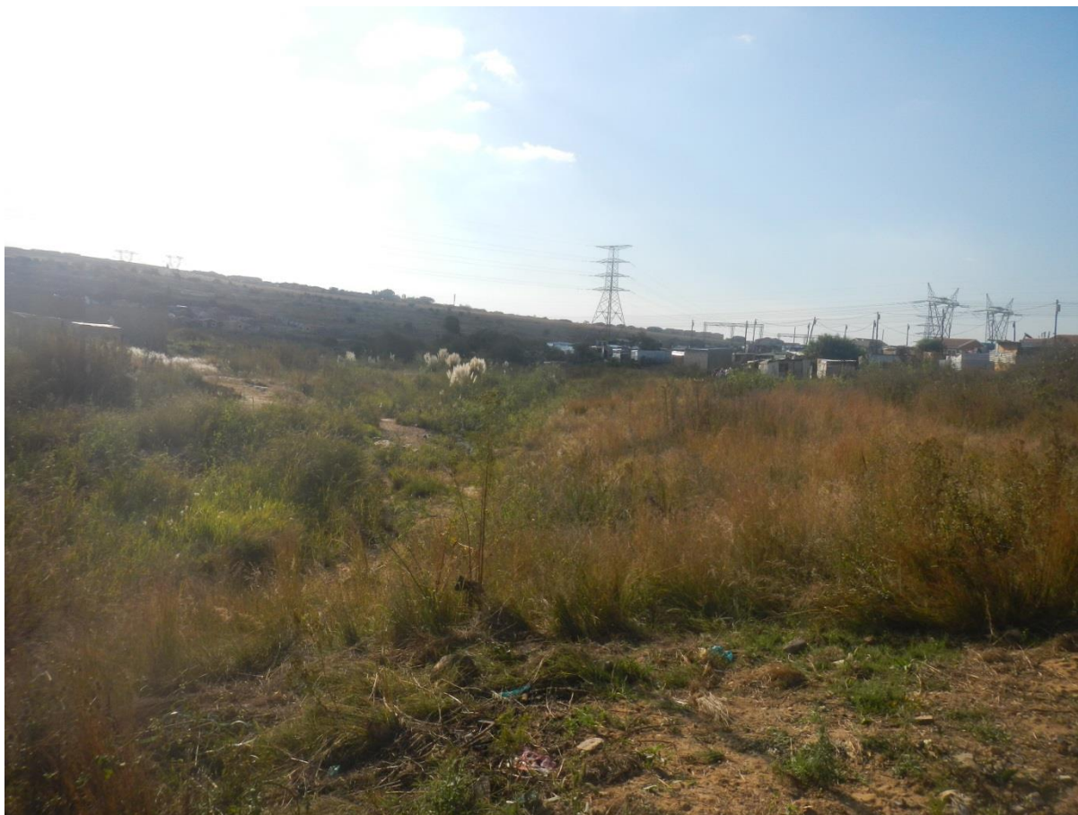
Figure 12: View of some of the power lines traversing across and along the proposed development site
