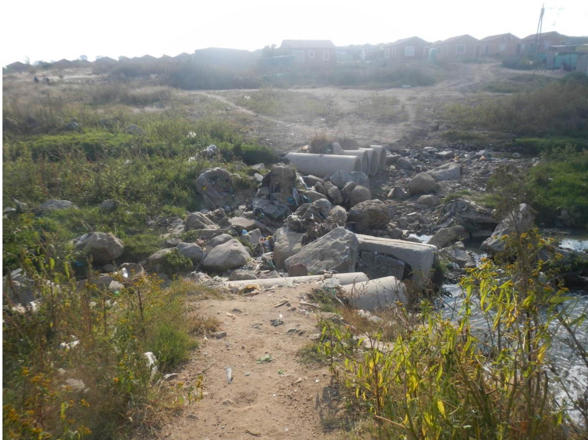
Figure 8: View of bridge one (1). Note the water pipers that were either meant for a proposed development or removed from an old development
