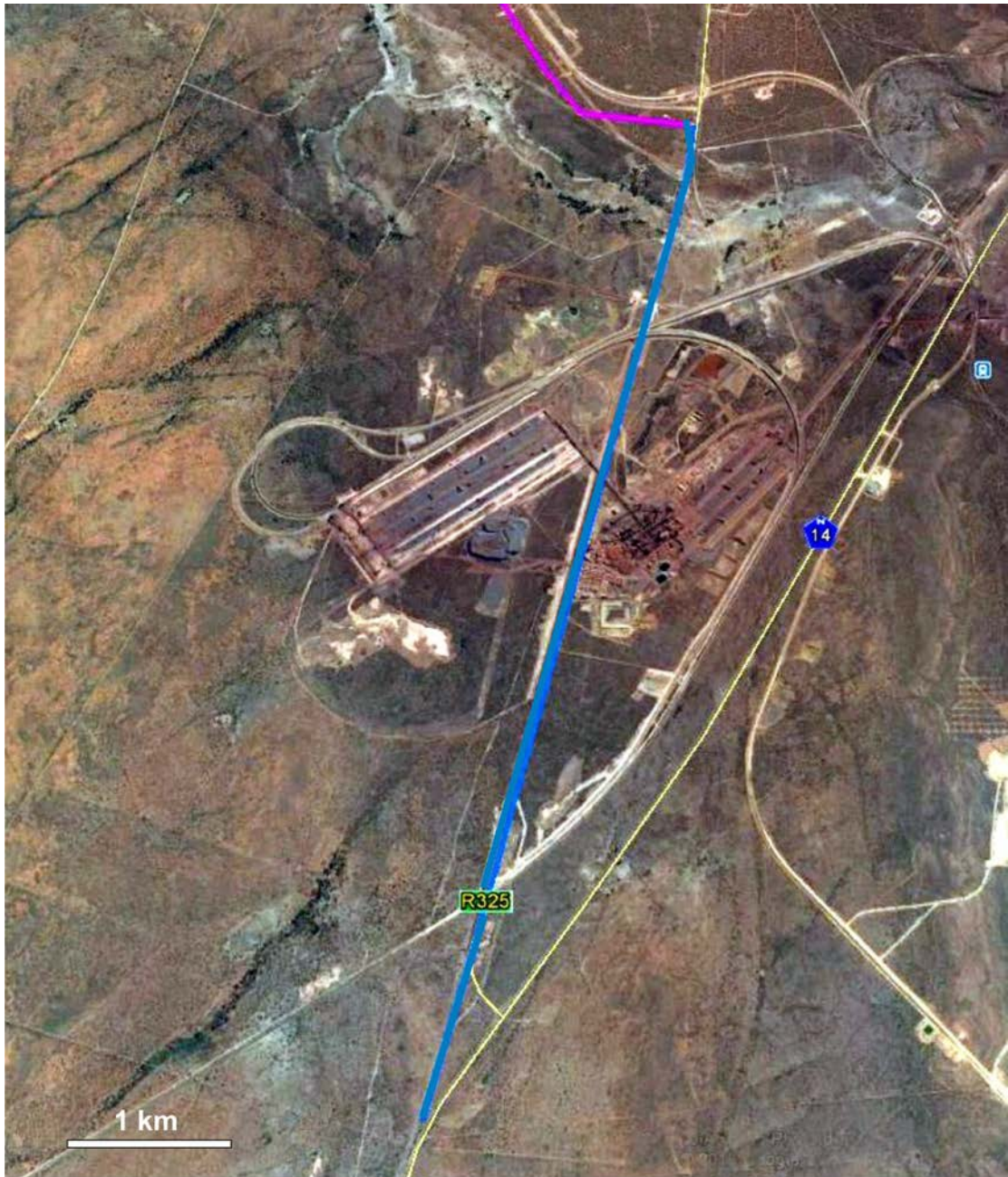
Figure 5. Aerial view of the pipe line section at Parson 564 and Gamagara 541. The pipe line will be placed directly adjacent and parallel to an existing line that runs directly next to the R325 road within an area that has been severely disturbed by earlier and ongoing mining activities.
