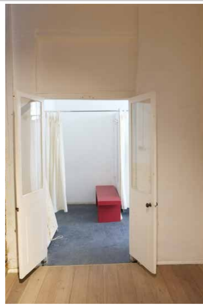
Figure 15. Ground floor, rear door
