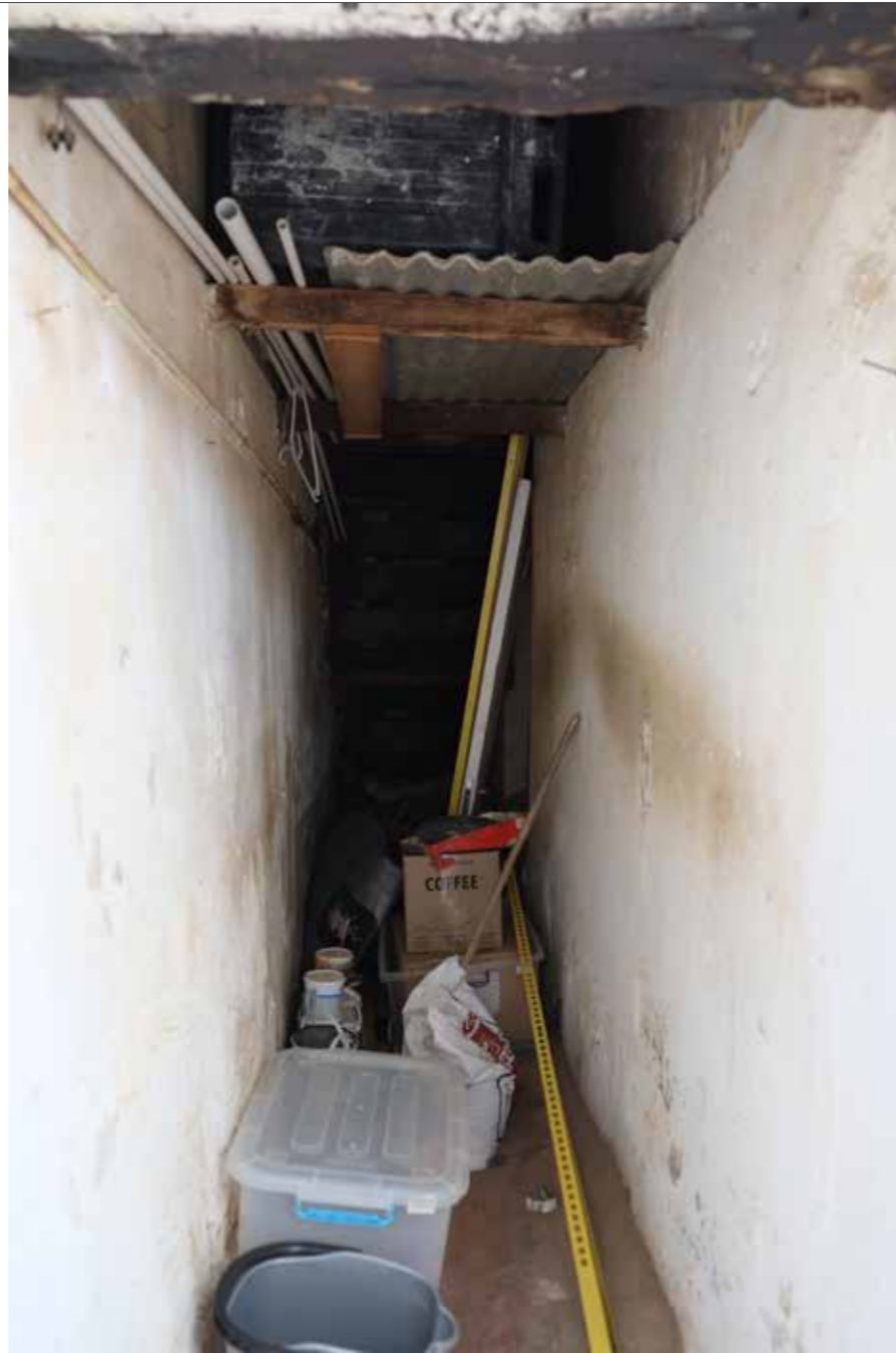
Figure 37. Ground floor, passageway beneath stairs
