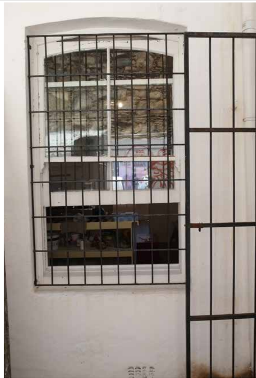
Figure 41. Ground floor rear window: arched top is an indicator of early stone construction (shallow arched stone lintel in place of rare timber). Wide vertical sash window in frame is almost flush with external wall suggesting is early (pre-c1815) Cape Dutch design
