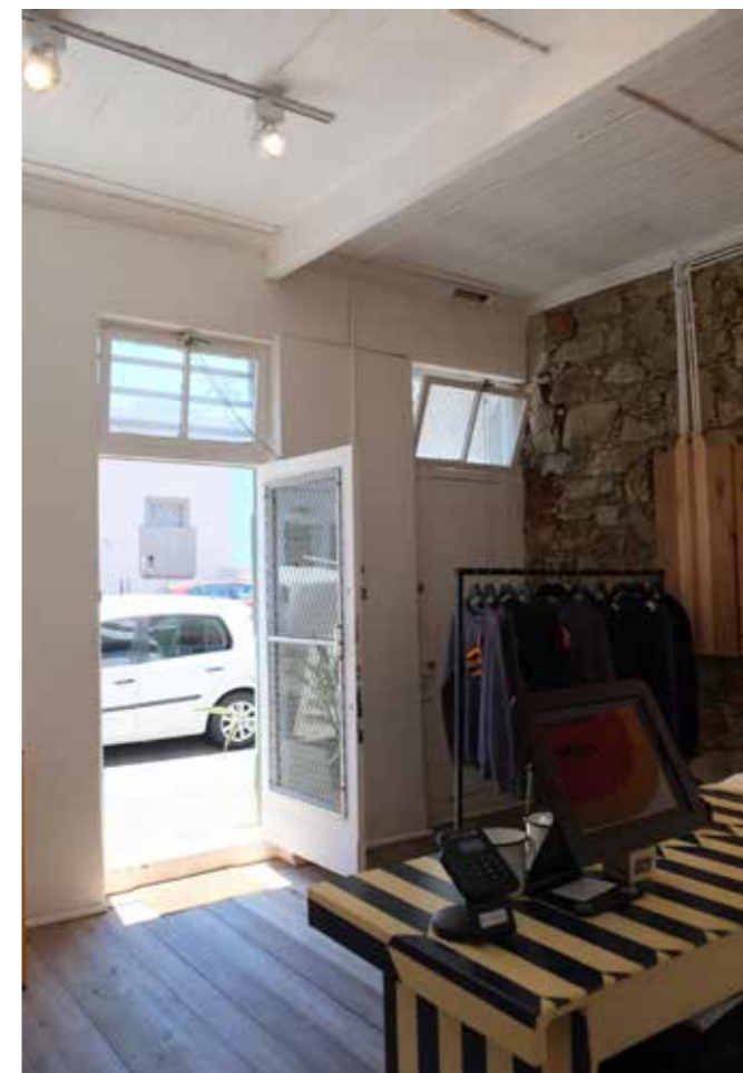
Figure 8. Ground floor showing two entries with beam suggesting earlier partition wall
