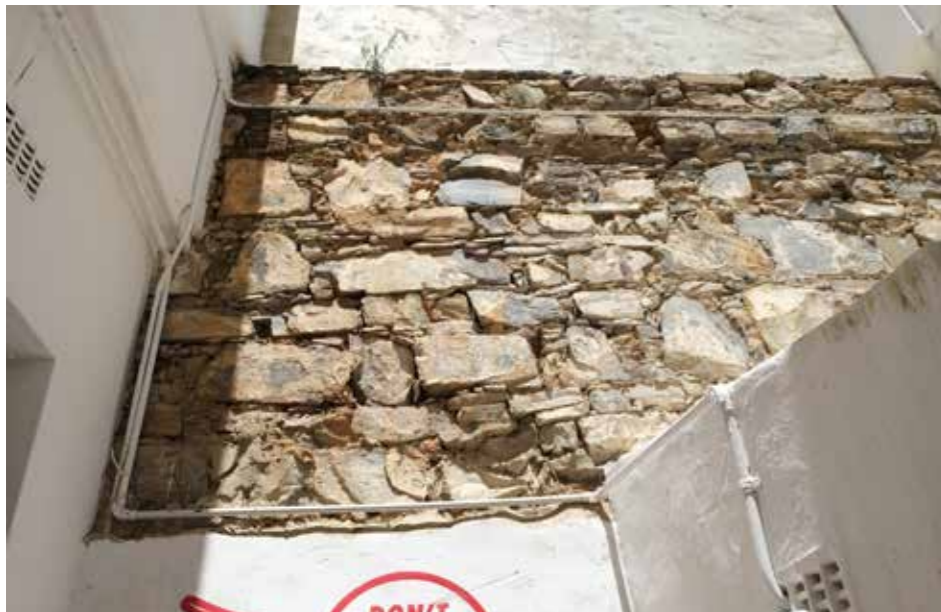
Figure 39. Ground floor view of rear shared courtyard wall
