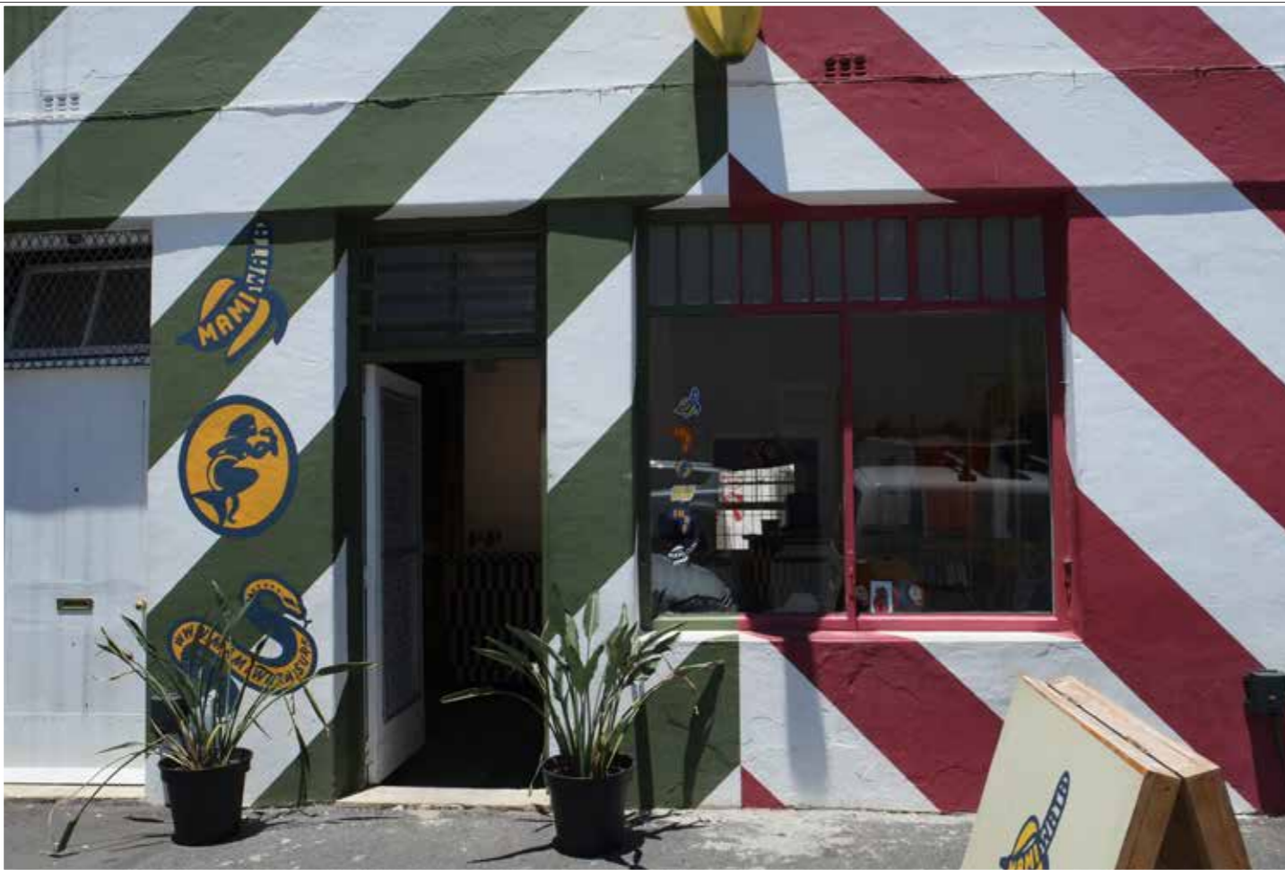
Figure 5. Ground floor: two north entries to front room and non-original window.
