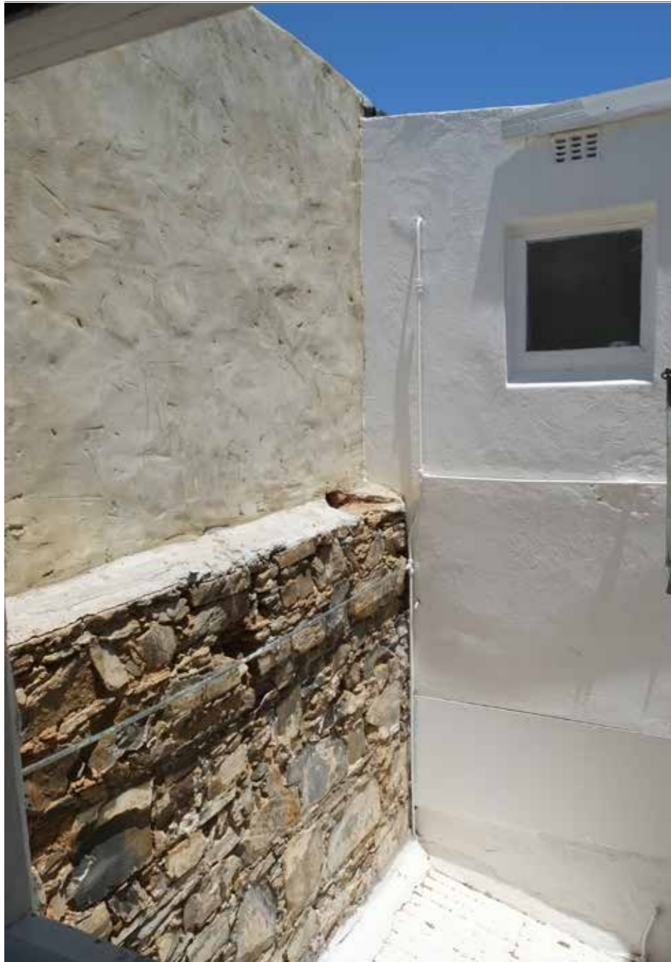
Figure 36. First floor view of courtyard rear shared wall
