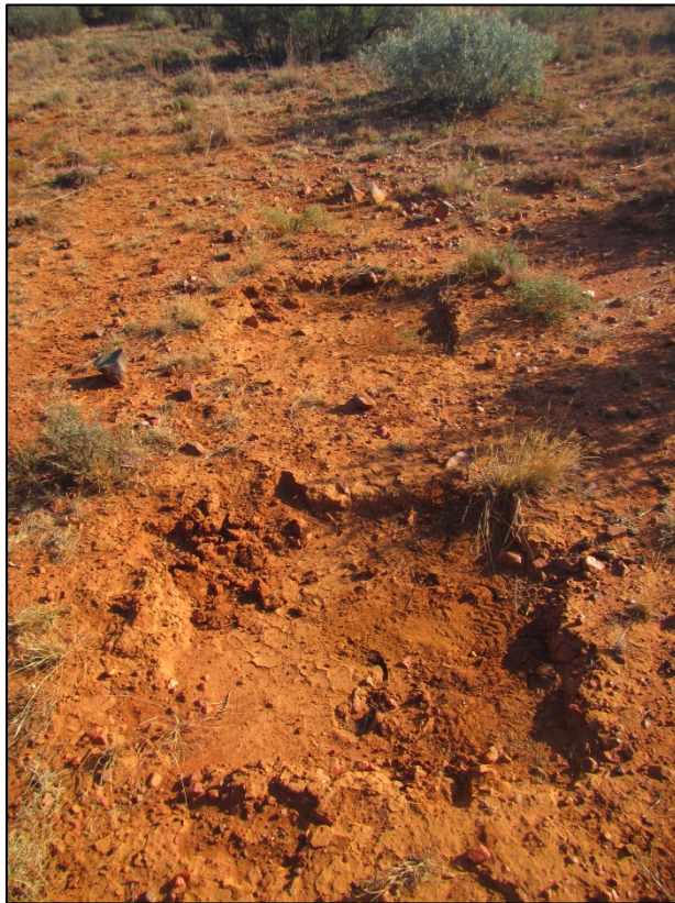
Figure 8 – Remains of previous mitigation work still visible on the day of the monitoring
