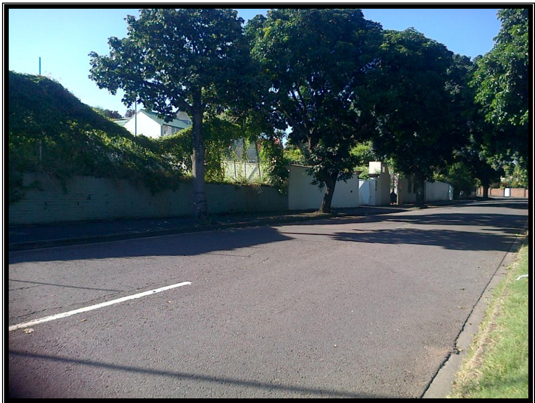
STREET ELEVATION FROM PROBLEM MKHIZE ROAD
