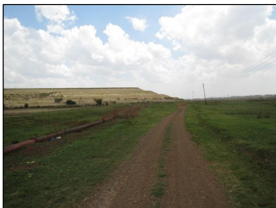
Figure 6 – View of beginning of Rooikraal pipeline at the base of the Rooikraal TSF that
