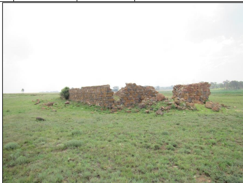
Figure 22 – View of the structure at ROK030
