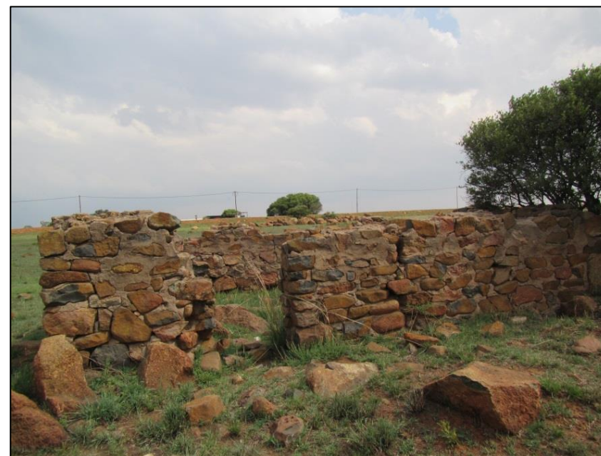
Figure 21 – One can see the relatively good preservation of the structure
