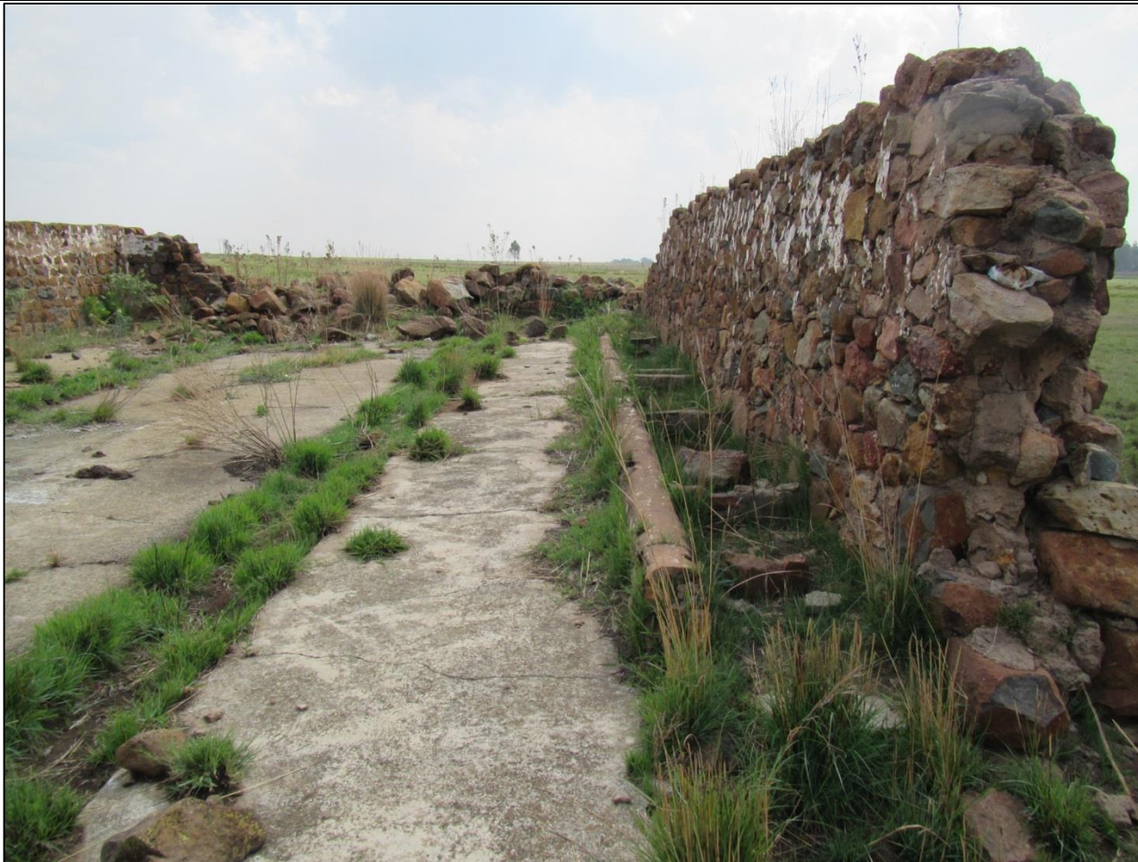
Figure 24 – One can see the feeding trough running along the inner edge of the wall
