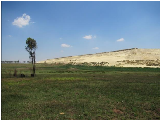
Figure 4 – View of TSF in background more or less undeveloped land in foreground
