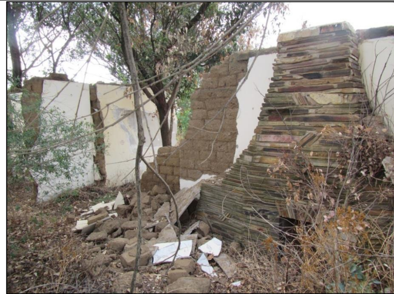
Figure 16 – Interior view of one of the rooms of the man homestead
