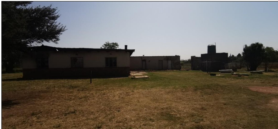
Figure 56 - Site VDB04, which is an intact but abandoned structure. The structure consists of brick, concrete, and a zinc roof. Apart from the main structure, there is another smaller structure as well as a small square structure with a water tank (Jojo) on top.
