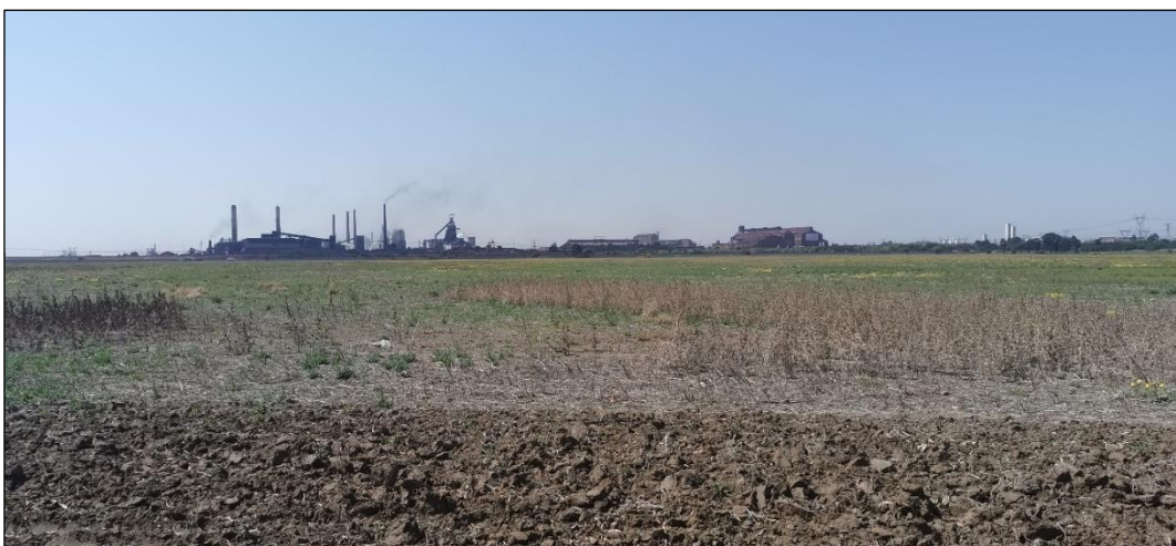
Figure 32 - General view of the AMSA industrial works in the distance.
