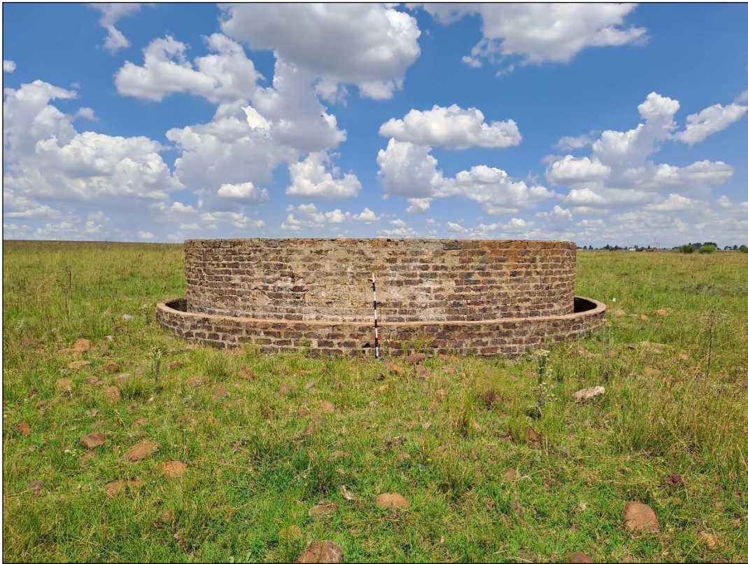
Figure 37 - Round reservoir made up of brick and concrete within the AMSA – 5 area.
