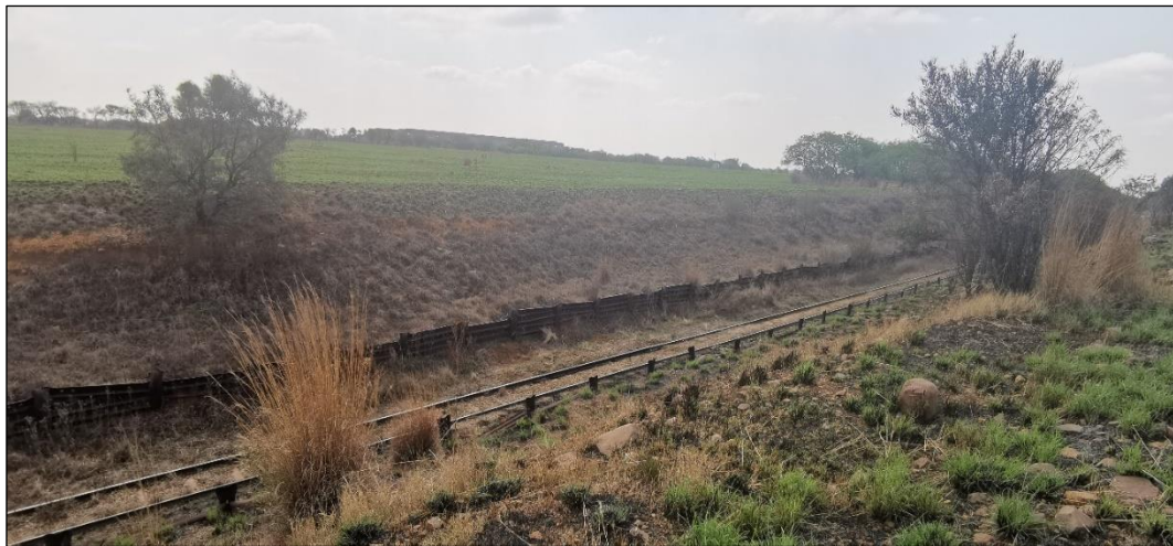
Figure 8 - View of railway tracks within the AMSA works area.
