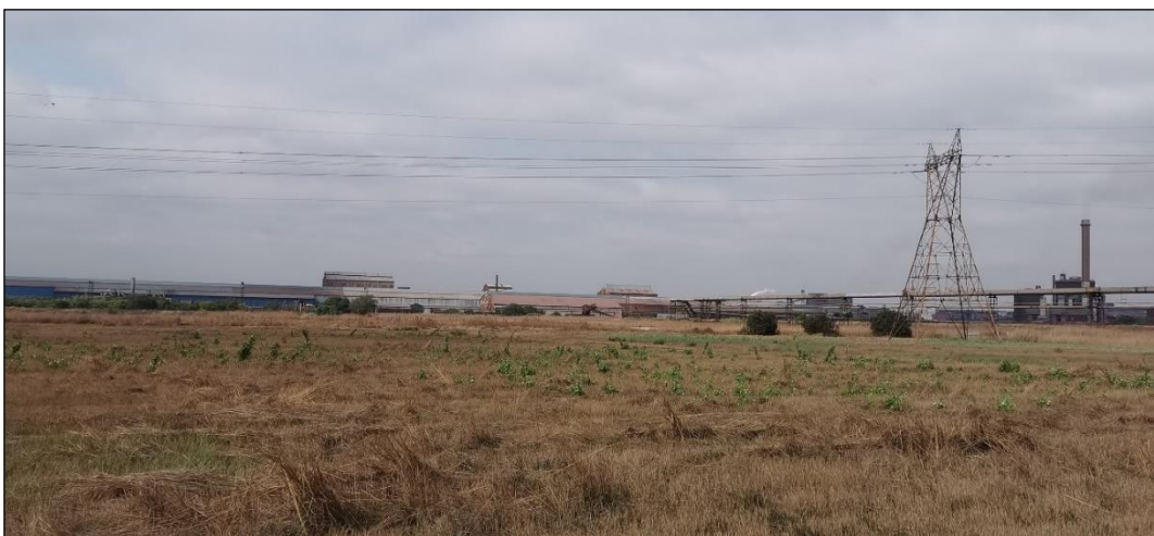
Figure 9 - General view of the powerlines located within the AMSA works area.
