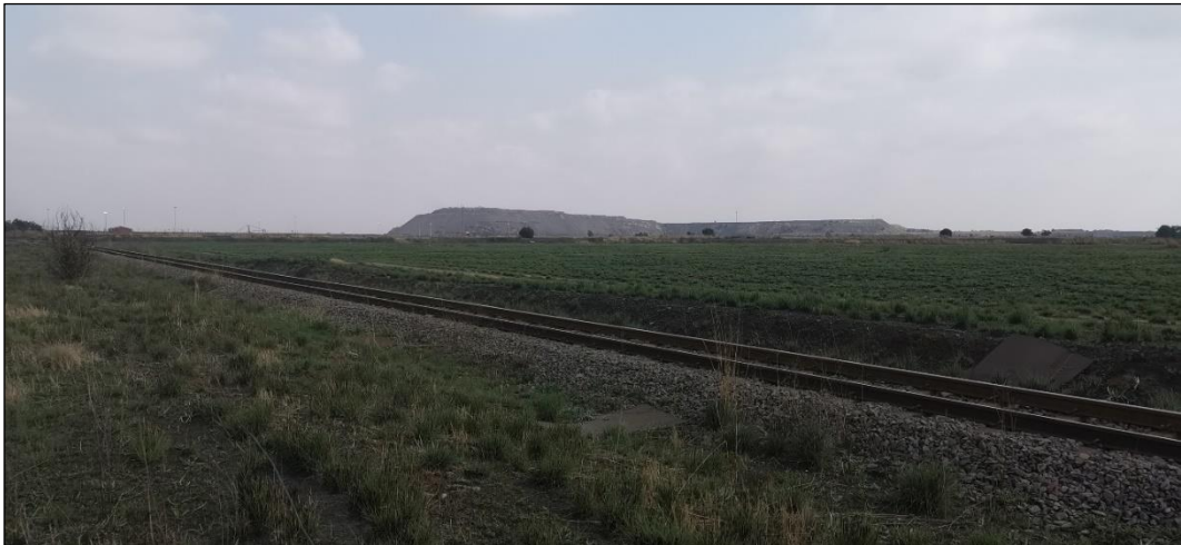
Figure 7 - View of railway tracks located within the AMSA works area.
