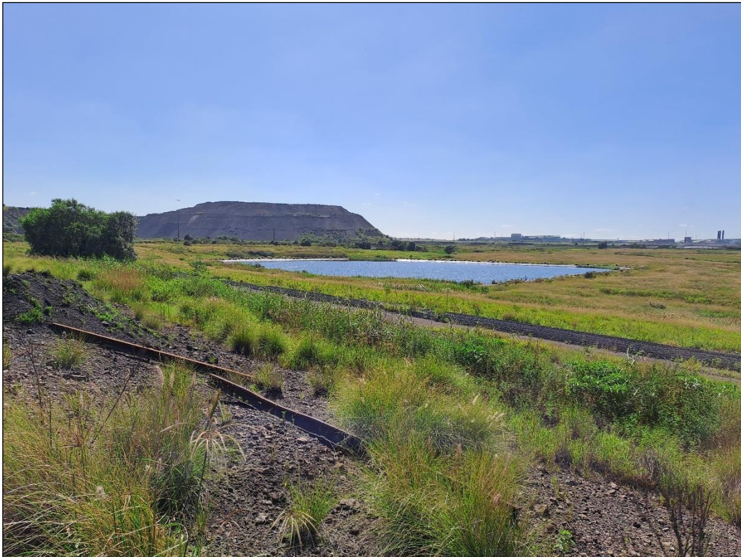
Figure 35 - Man-made dam located inside the AMSA works.
