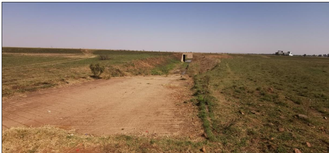
Figure 31 - General view of a service road that goes underneath the R554 national road, located in the AMSA – 3 area.
