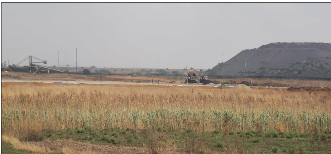
Figure 12 - Site clearing activities within the AMSA works area.
