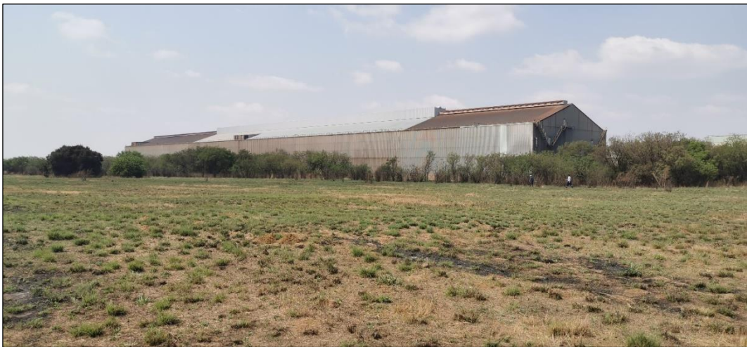
Figure 6 - Large building located within the AMSA works area.
