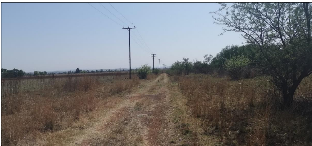
Figure 29 - General view of telephone lines located in the AMSA – 3 area.
