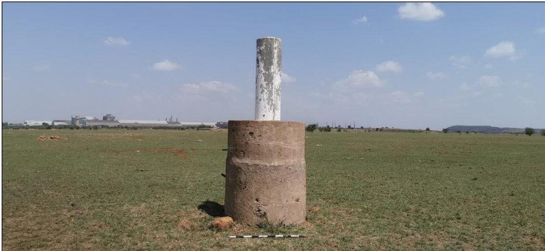
Figure 57 - Site VDB02 is a historical trigonometrical beacon (no 566). The beacon is located in a flat open field and consists of concrete and white paint.
