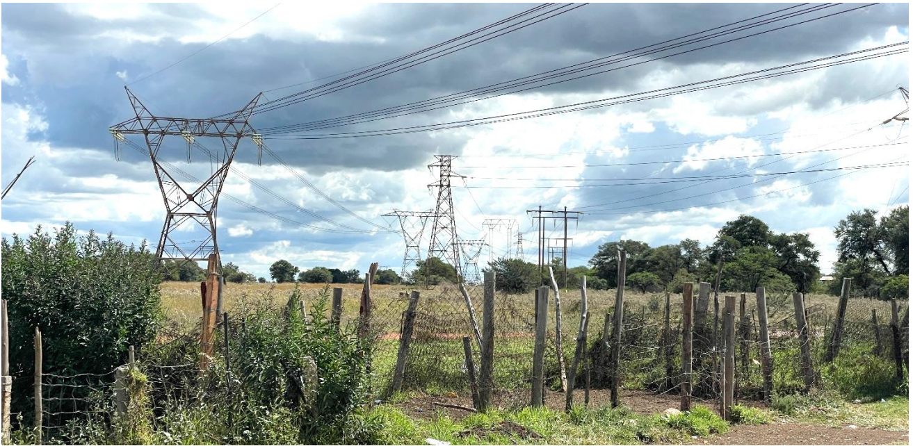
Figure 8: Example of the existing power lines crossing the site
