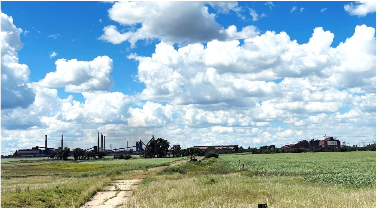
Figure 4: ArcelorMittal Vanderbijlpark Plant located adjacent to the proposed AMSA Vanderbijlpark PV Solar Facility.
