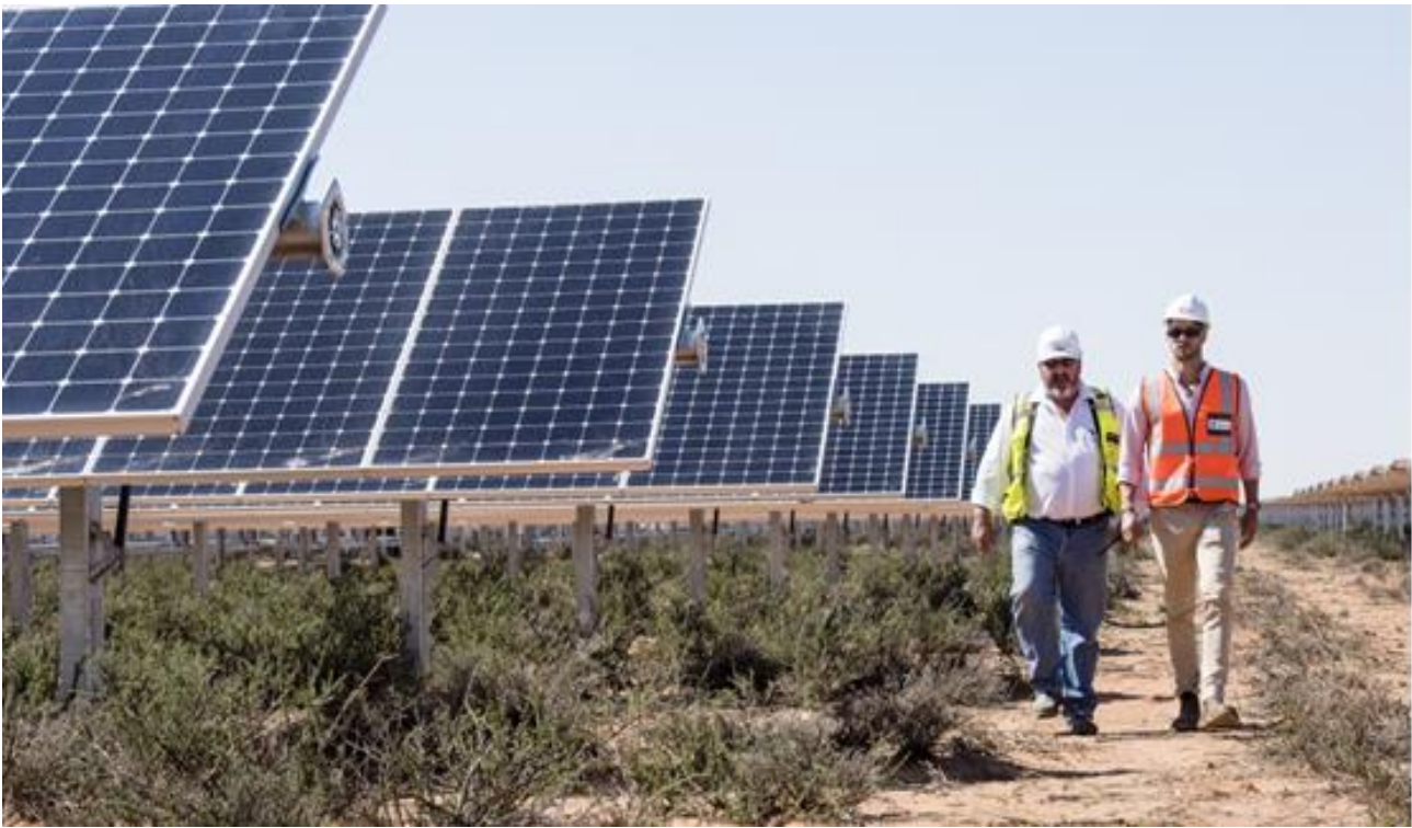
Figure 1: Photovoltaic (PV) solar panels. (Photo: SunPower Solar Power Plant- Prieska)
