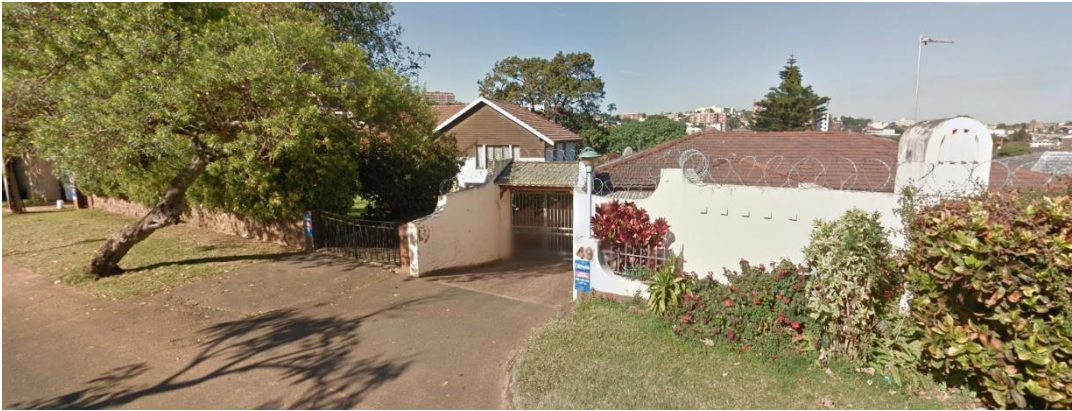
Image 25. Image of Properties opposite to the road ERF 71/230 and ERF 71/230 2009 (From Google Map)
