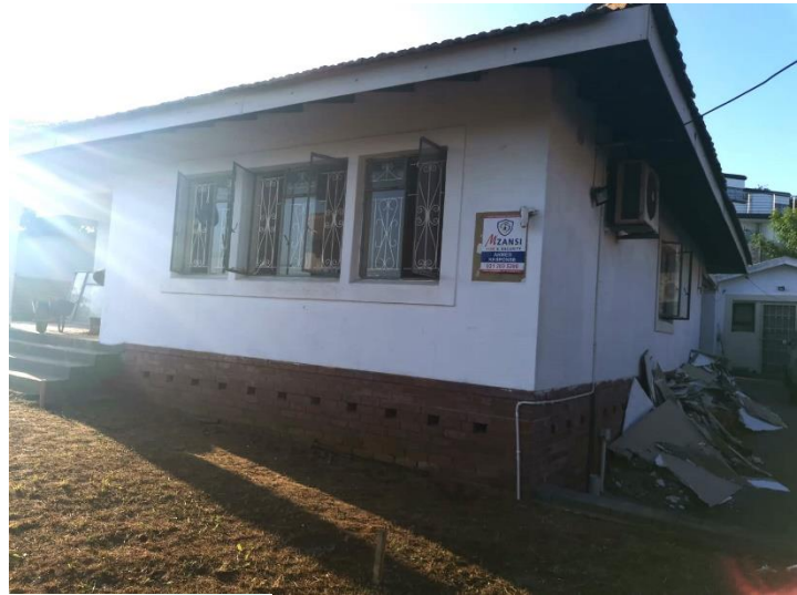
Image 11. Image of the Front House (First Site Visit)
