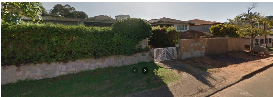
Image 22. Image of the Front House with Property adjacent ERF 39/230 2013(From Google Map)
