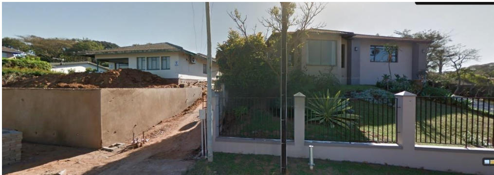
Image 18. Image of the Front House with Property adjacent ERF R37/230 2013(From Google Map)
