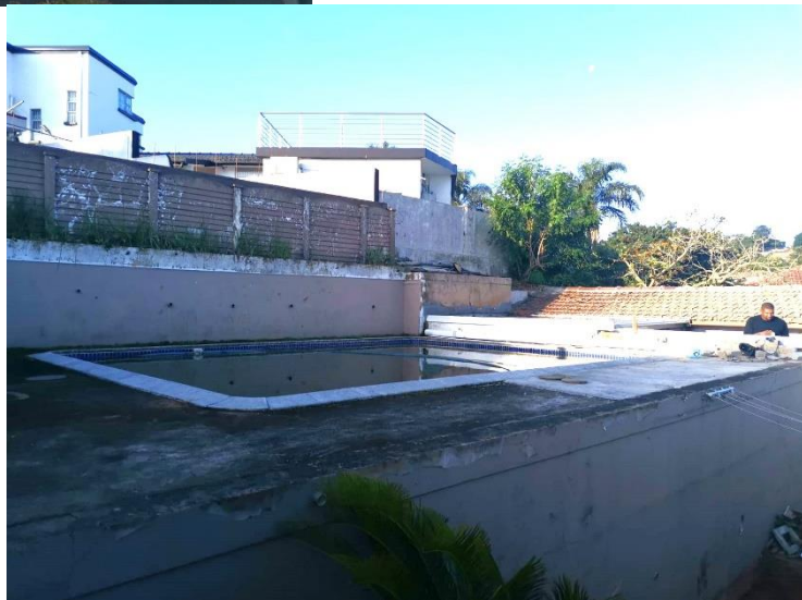
Image 13. Image of the Pool (First Site Visit)
