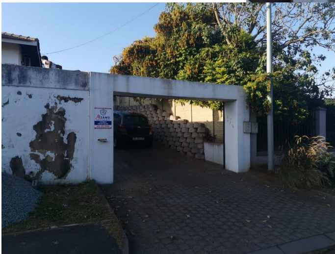
Image 15. Image of the Drive way access South elevation (First Site Visit)
