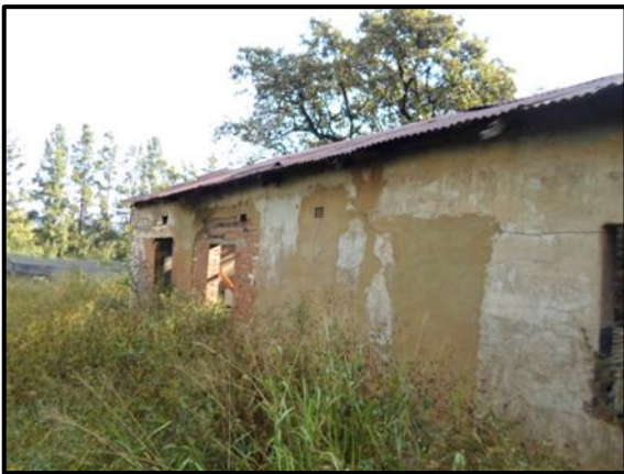
Figure 8.8. Structure at GG003.
