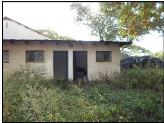
Figure 8.9. Structure at GG003.
