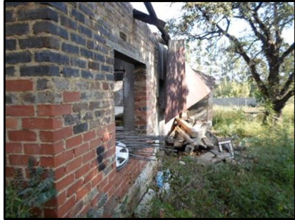
Figure 8.7. Structure at GG003.
