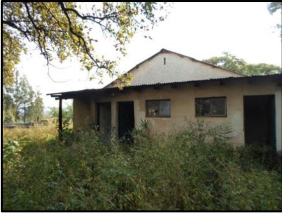
Figure 8.6. Recorded structure at GG003
