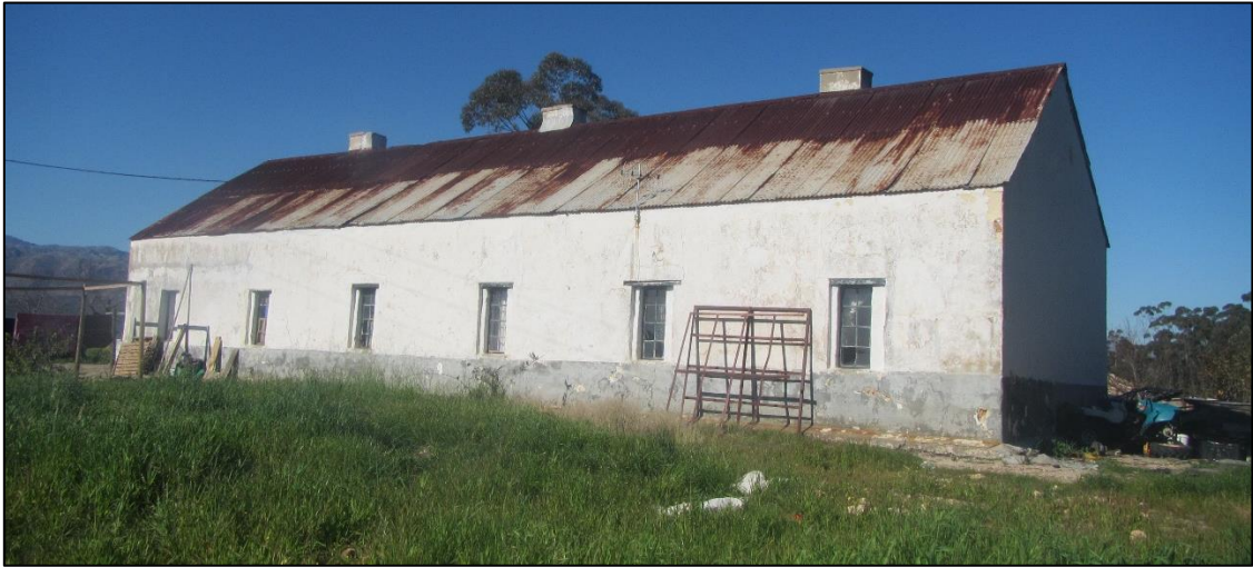
The north-western façade of the existing cottage on site.
