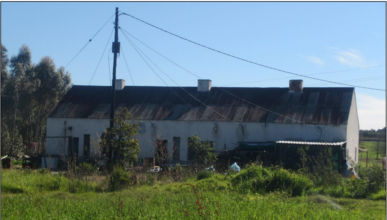
The south-eastern façade of the existing cottage on site.
