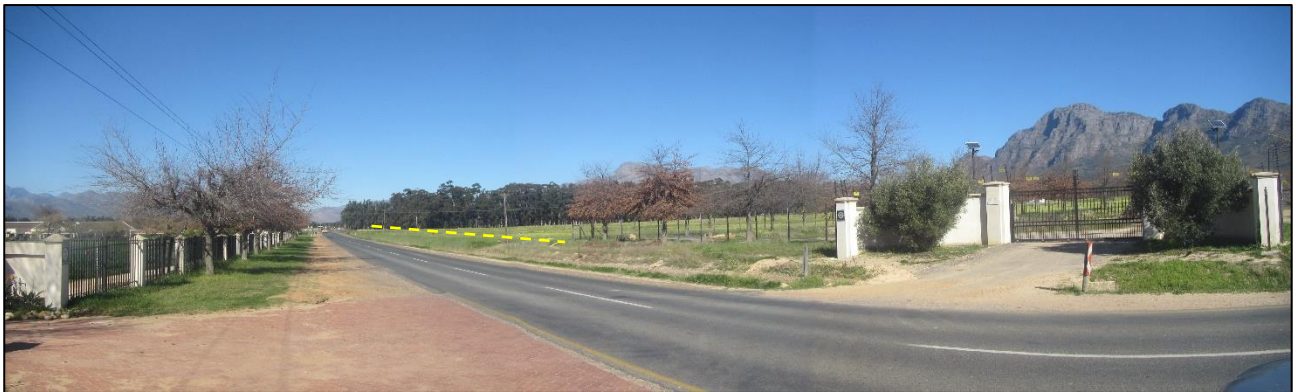
View towards the southeast along the MR205 showing the neighbouring fenced properties. The yellow dashed line indicates the road edge of the site to be fenced (although the actual property includes the adjacent strip of road).
