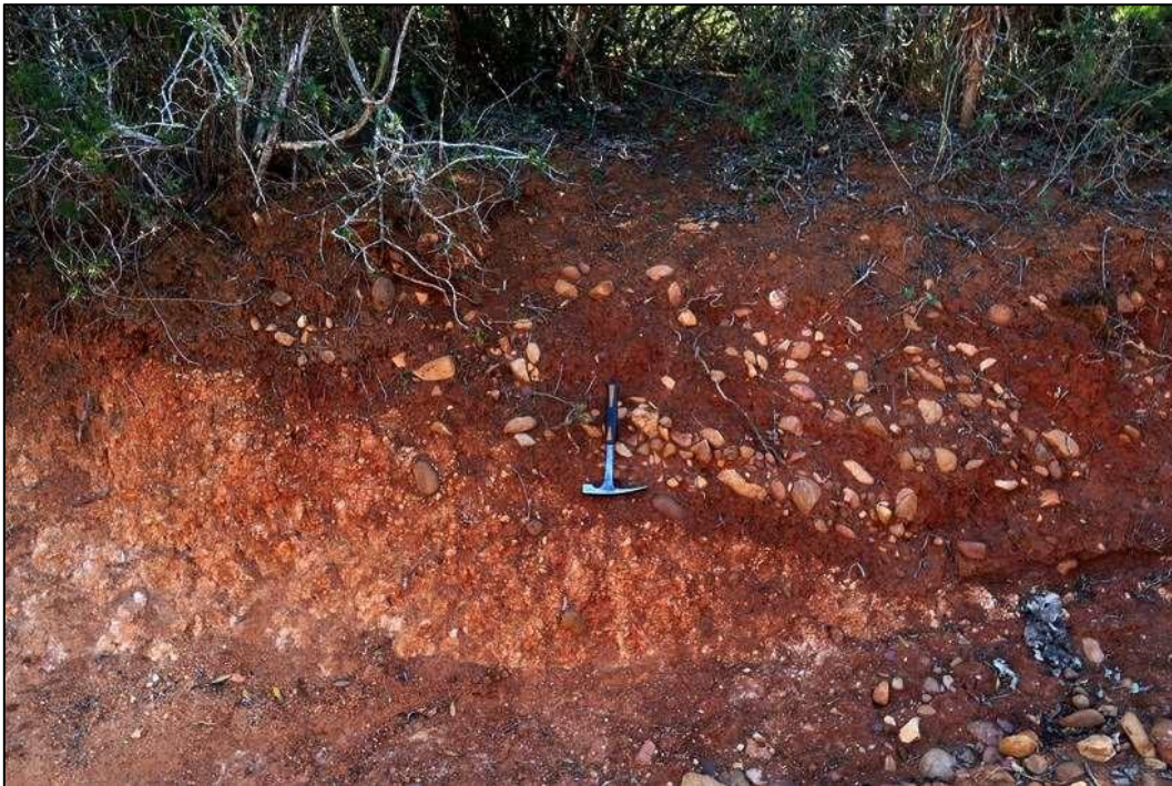
Figure 14: Road cutting on the SW margins of the Grassridge Plateau showing Alexandria Formation calcarenites overlain by deeply rubified soils and pebbly concentrations of the “Bluewater Bay Formation”, essentially a downwasted (eluvial / relictual) weathering product of the underlying unit (Hammer = 30 cm).
