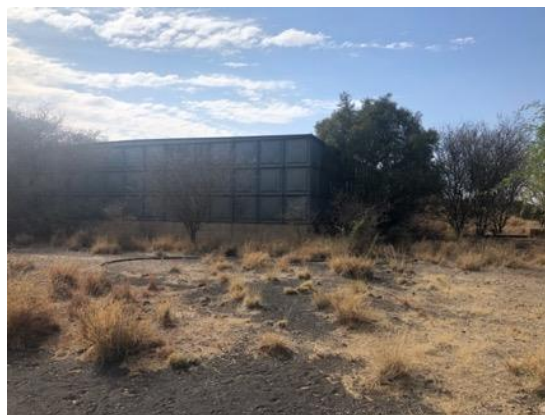
Figure 13 – Existing water reservoir at Middelpplaats Shaft
