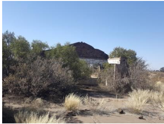
Figure 15 – Mining infrastructure in the proposed rail loop area
