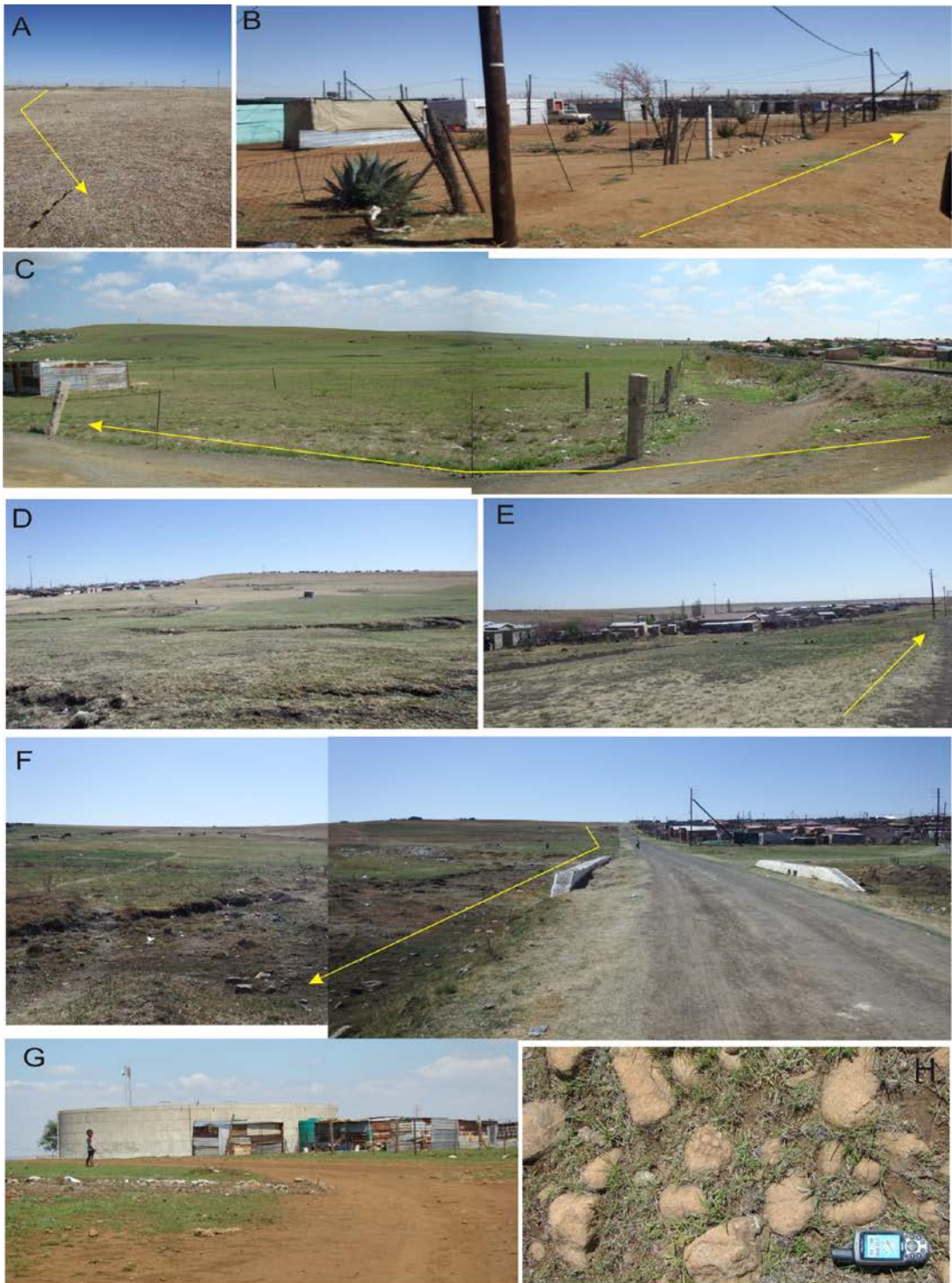
Figure 9. From the Frankfort WTW the pipeline runs adjacent to the R26 (A) and then divert east to follow an existing gravel road (B, C) in a northwesterly direction within the Namahadi township (D - F) where it passes the Namahadi Reservoir (G) and terminates at the northwestern boundary of the township. The footprint is completely underlain by dolerite intrusions (H).
