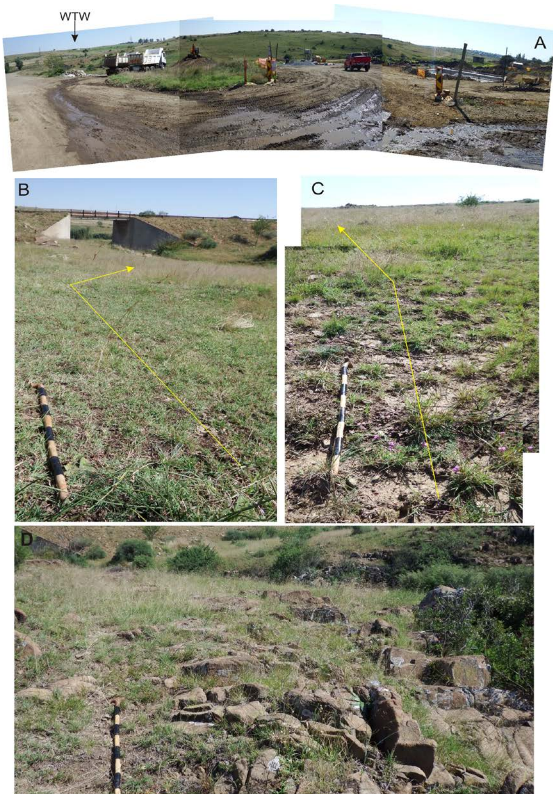
Figure 6. From the proposed new pump station site (A) the pipeline crosses a small tributary of the Wilge River at J.J. Hadebe Street (B) and then follows the road for about 100 m in a northerly direction (C) all underlain by dolerite intrusions (D).
