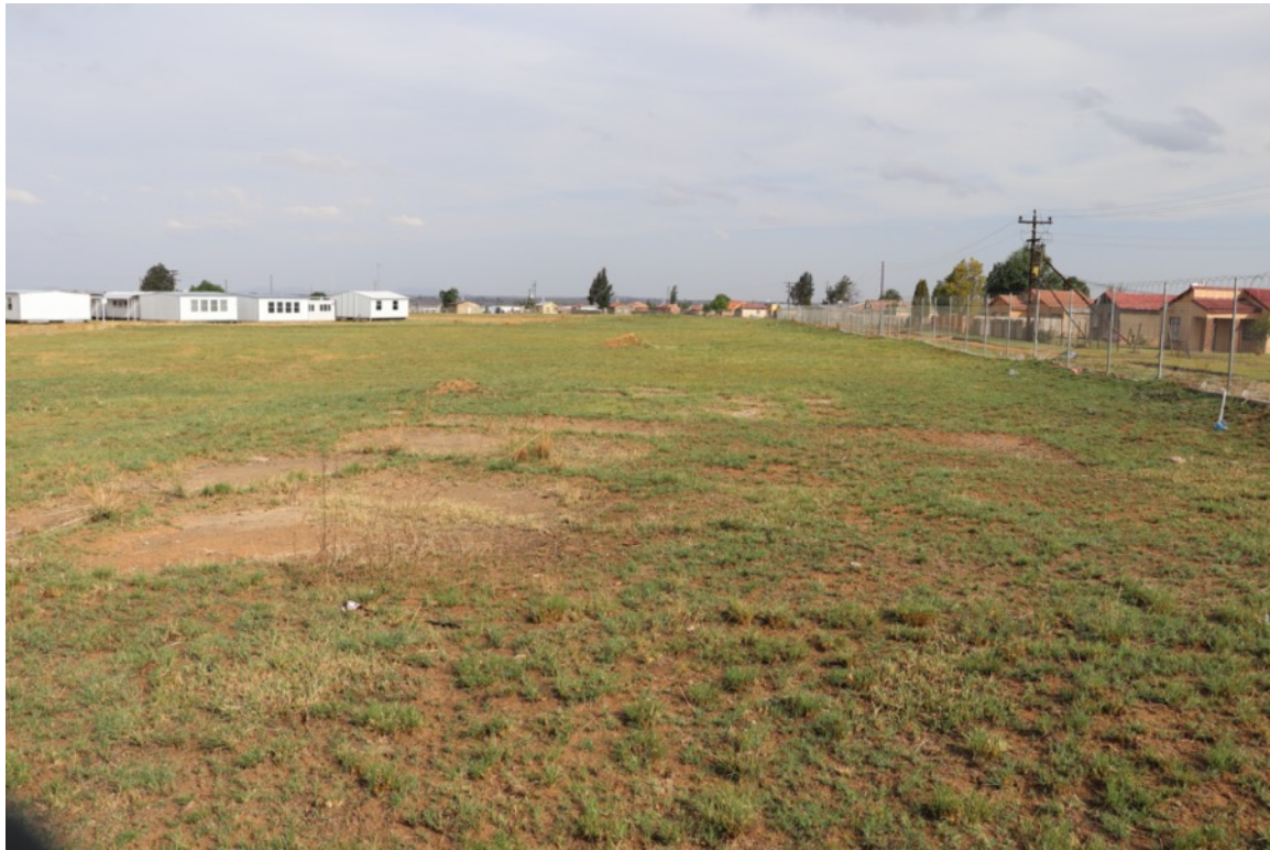
Figure 8 – View from the north towards the school buildings with fence visible on the right
