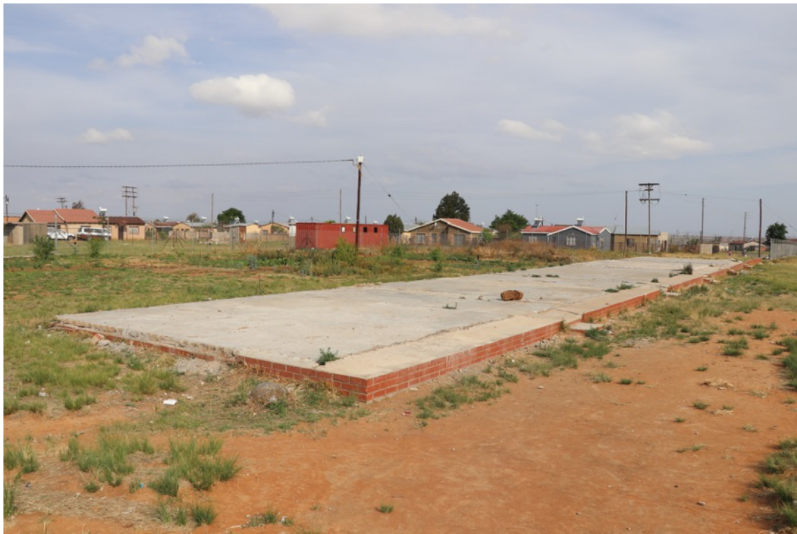
Figure 6 – Foundation of prefabricated building
