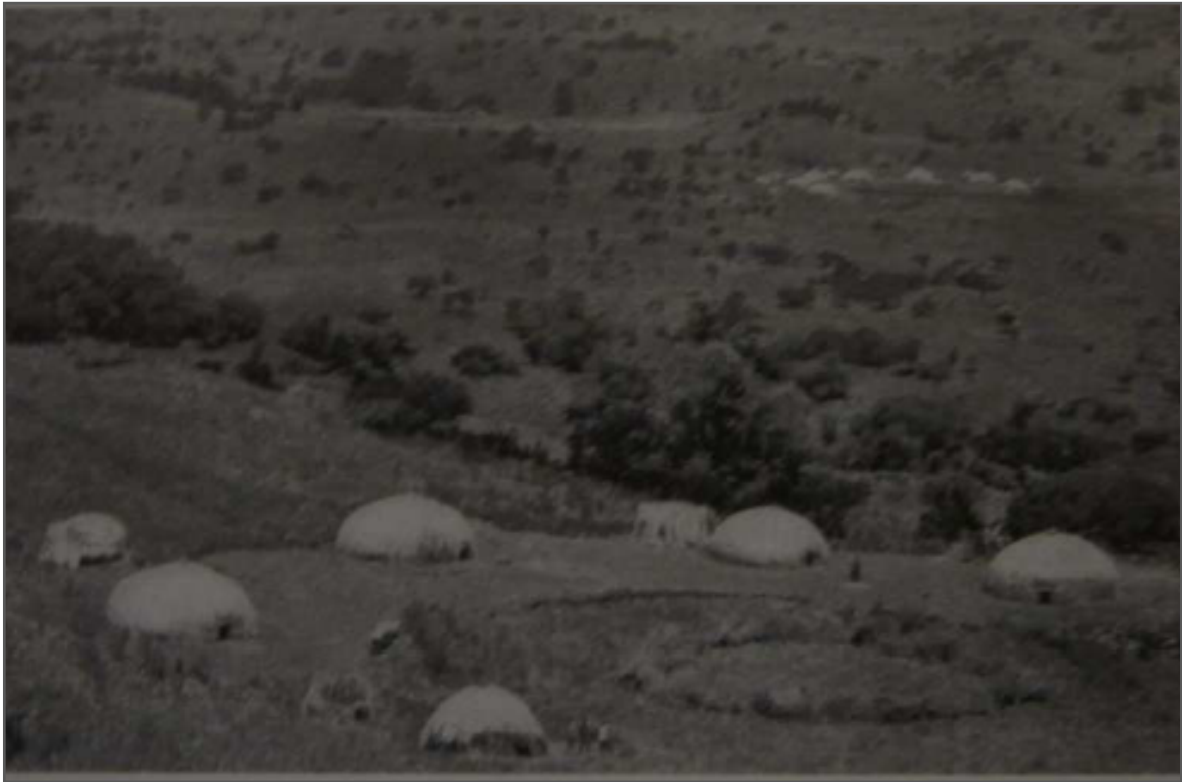
Figure 14- Pre-industrial Zulu village: beehive huts, note homestead built using thatch material (Colonial period picture) (Laband & Thompson, 2000)
