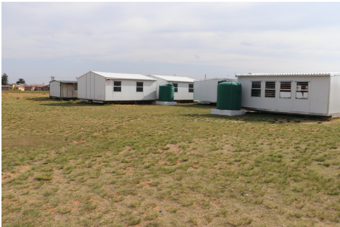
Figure 7 – View of the eastern section of the current school buildings
