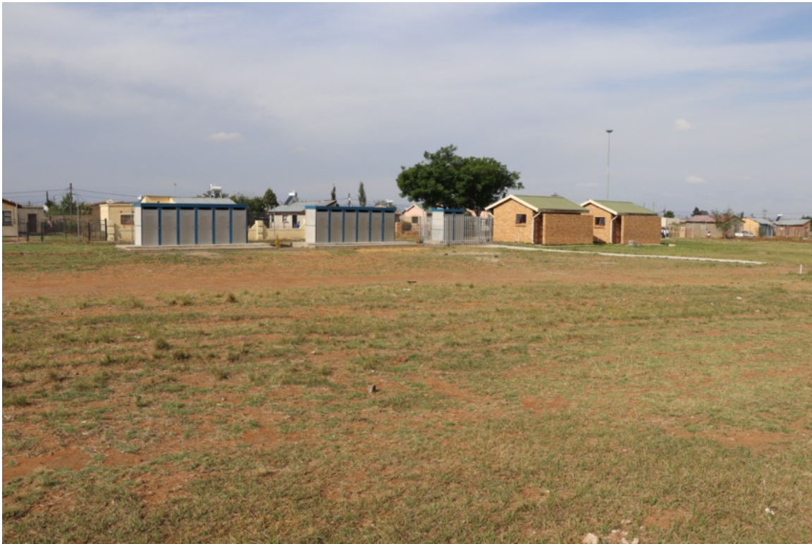
Figure 10 – Temporary and permanent ablutions
