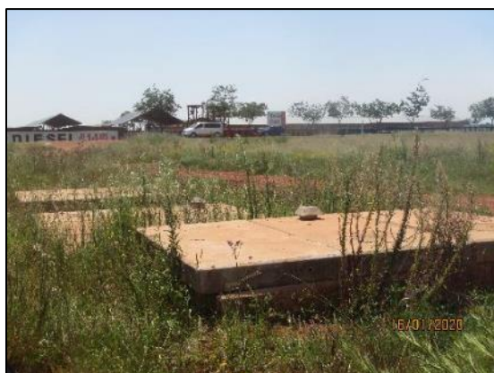
Figure 7 - Sewage pipelines located in south-western corner of project area
