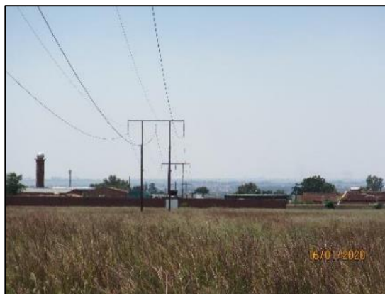
Figure 6 - Powerlines running through project area
