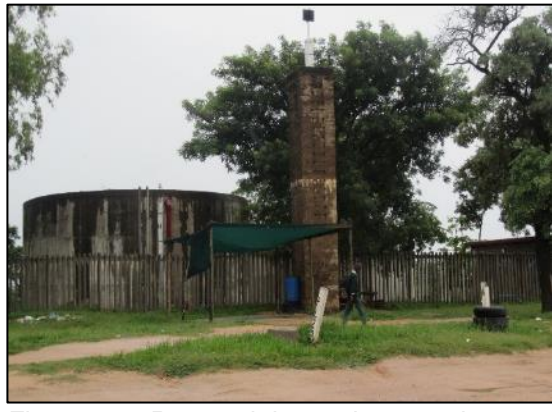
Figure 27 – Reservoir located next to the D4407 in Hluvukani
