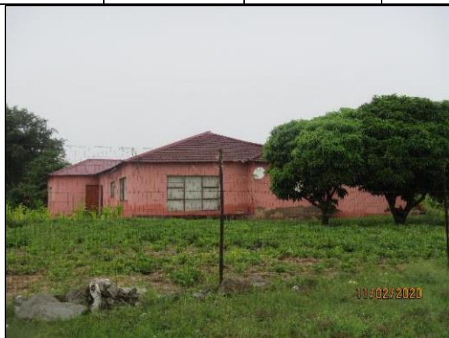
Figure 42 – View of HR-03 from the street
