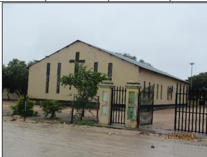
Figure 40 – View of Church
