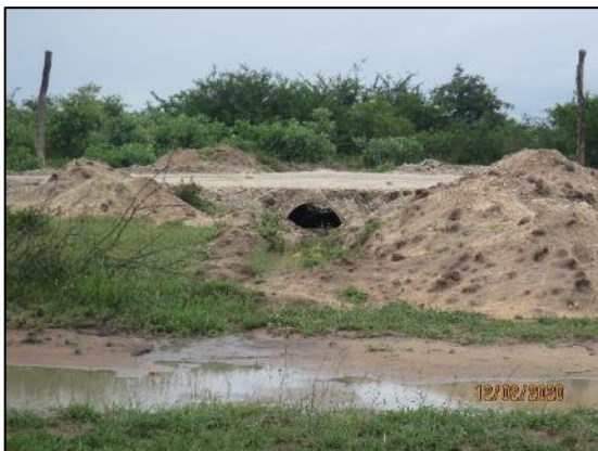
Figure 22 – Culvert 27 near Welverdiend
