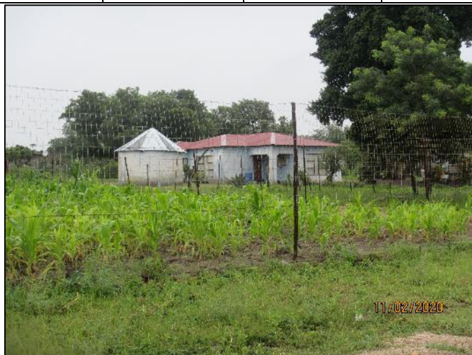
Figure 43 – View of HR-04 from the street
