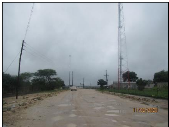
Figure 12 – View of the D4409 in Welverdiend
