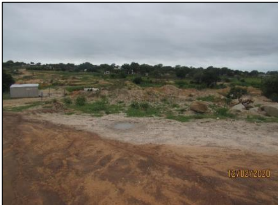
Figure 15 – Bridge construction site on the D4409 (View taken facing south)
