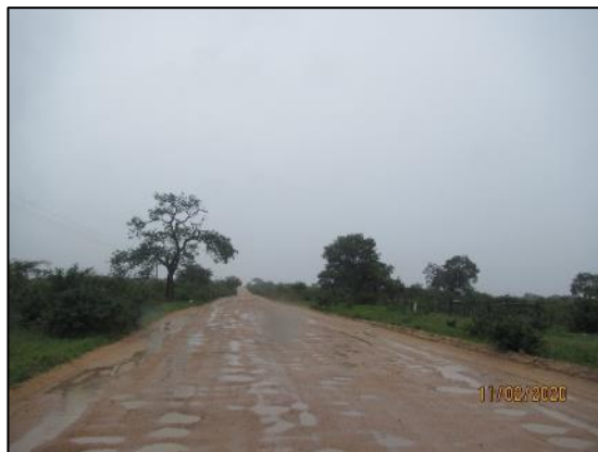
Figure 23 – View of the D4407 between Welverdiend and Hluvukani
