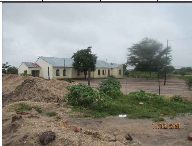
Figure 39 – View of Church
