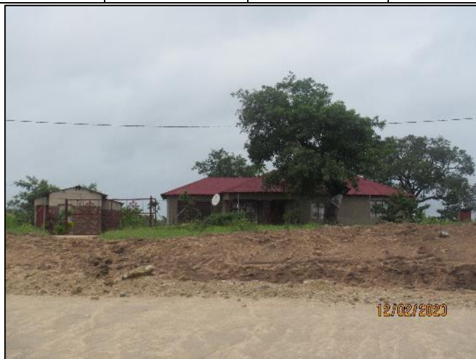
Figure 44 – View of HR-05 from the street
