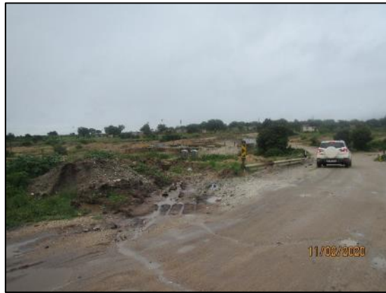
Figure 14 – Bridge construction site on the D4409
