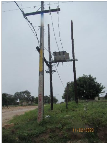
Figure 20 – Powerlines found throughout the project area
