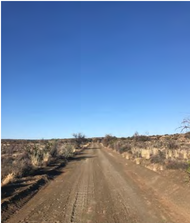
Figure 22: Main gravel farm road.
