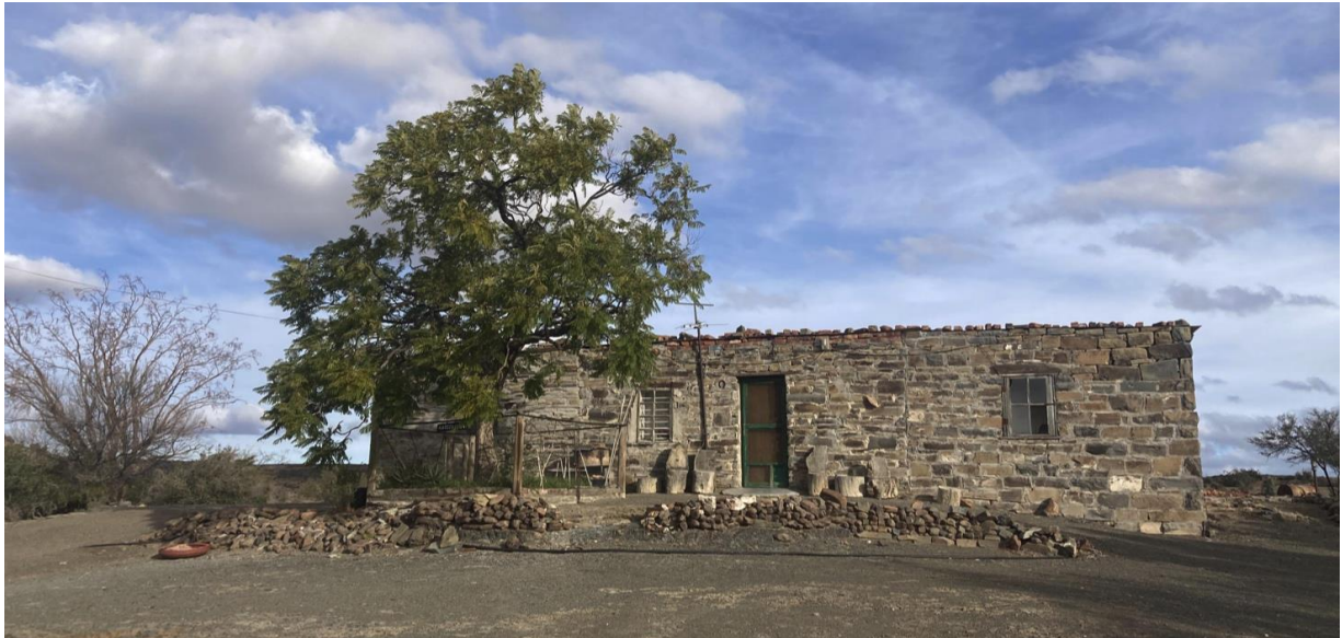
Figure 36: Kareerivier homestead front façade
