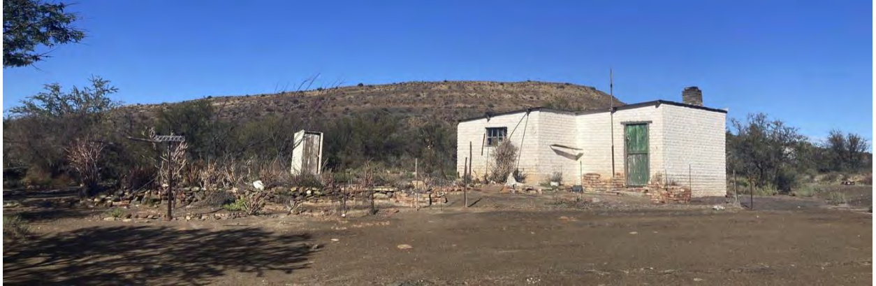
Figure 34: One of the currently inhabited Platdoorn homesteads with Platdoring se Kop behind.
