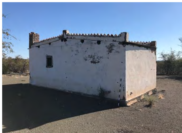
Figure 59: Back view of KO-01
