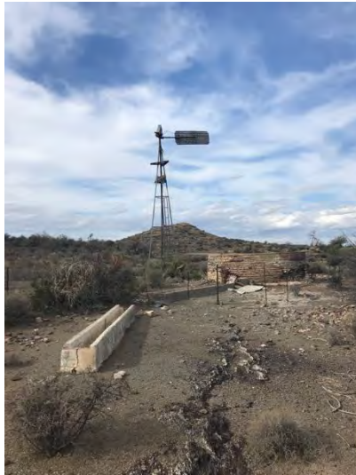
Figure 28: Example of dilapidated windmill and water trough.
