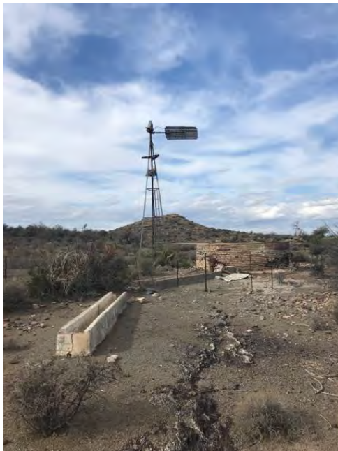
Figure 29: Example of dilapidated windmill and water trough.
