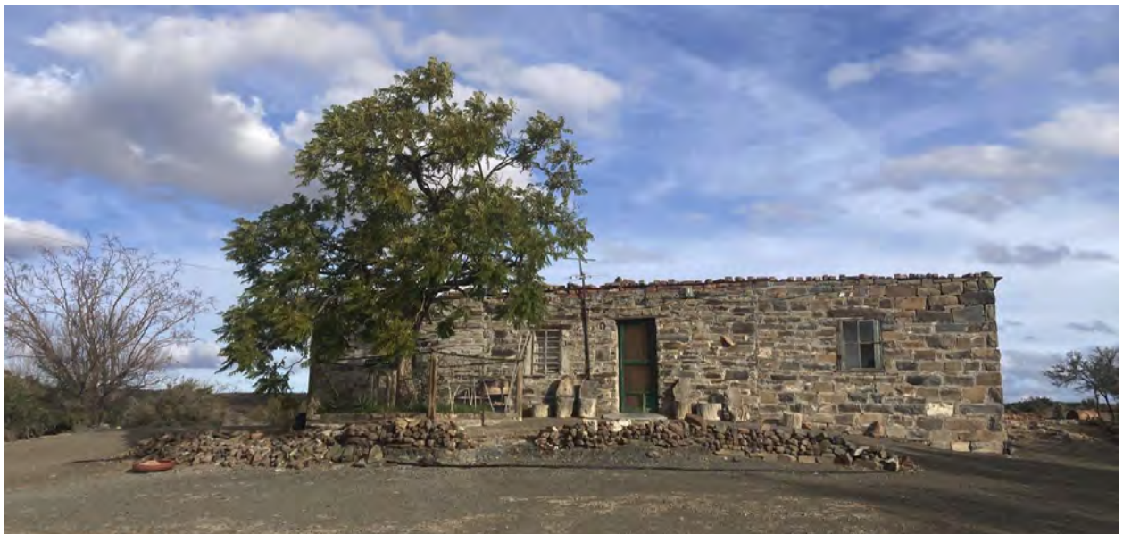
Figure 47: Kareerivier homestead front façade
