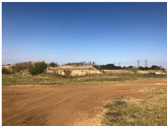
Figure 39 – Remaining structures of the power station infrastructure at KF009
