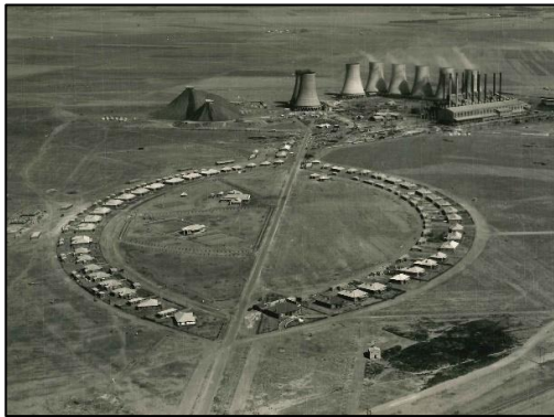
Figure 17- Aerial view of Klip power station with the residential houses still under construction
