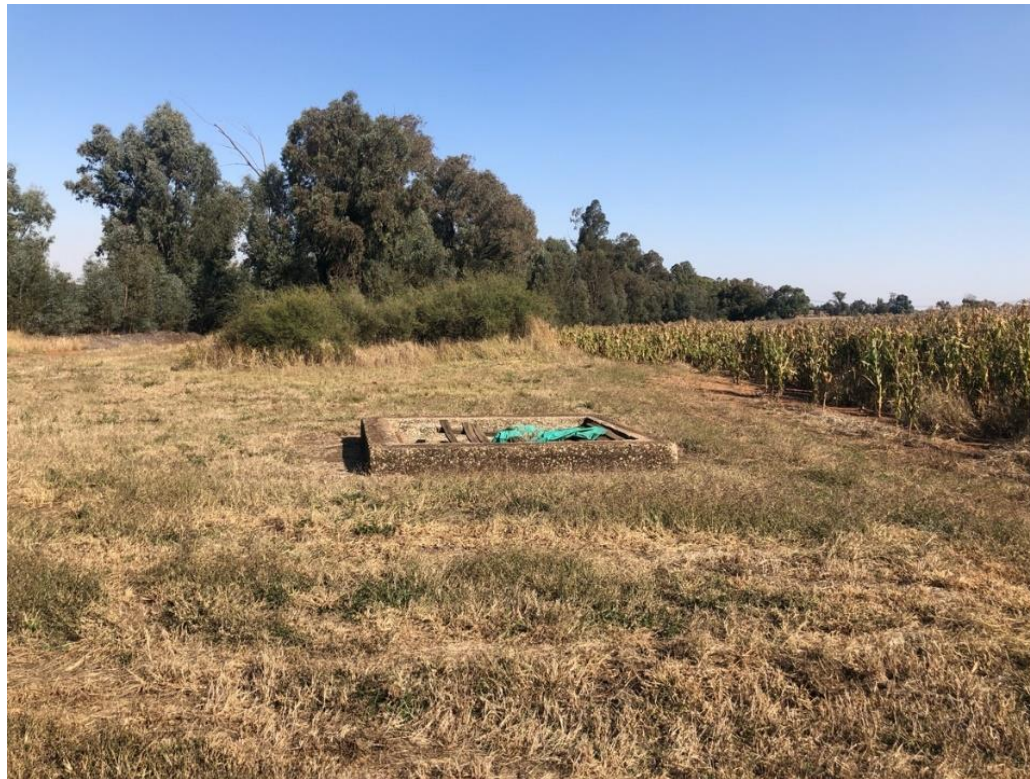
Figure 45 – View of the shaft collar of the vertical shaft at KF011
