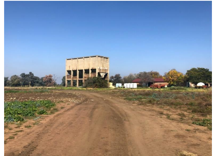
Figure 47 – The concrete coal tip of the Springfield Colliery west shaft
