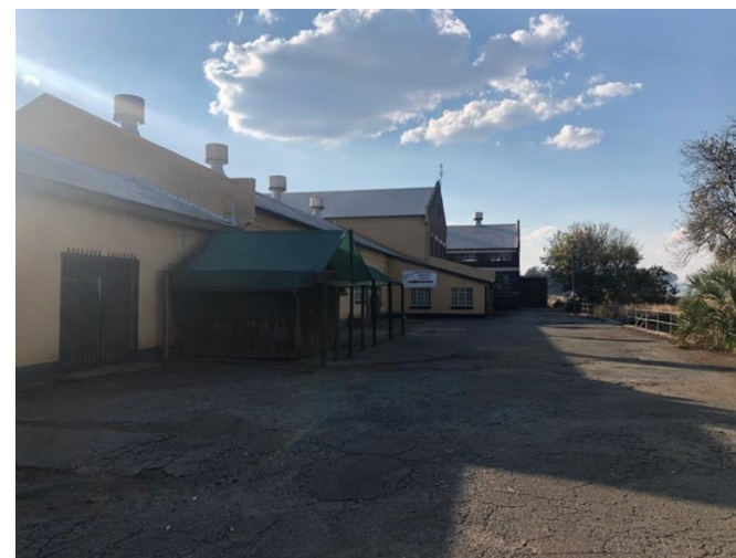
Figure 40 – The original workshops of the Klip power station at KF012
