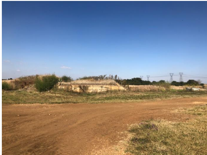
Figure 40 – Remaining structures of the power station infrastructure at KF009
