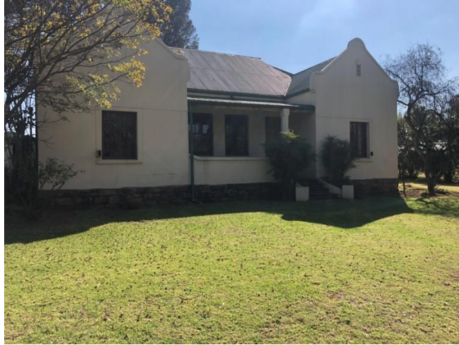
Figure 34 – Front façade of the main house
