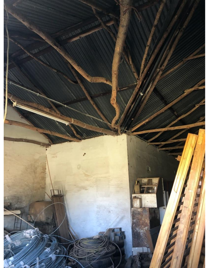
Figure 39 – Interior view of the waenhuis with the decorative wooden beam hiding the steel trusses
