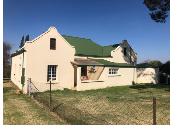
Figure 35 – View of the back of the house, note the steel framed windows and lean-to roof addition
