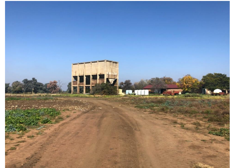
Figure 48 – The concrete coal tip of the Springfield Colliery West shaft
