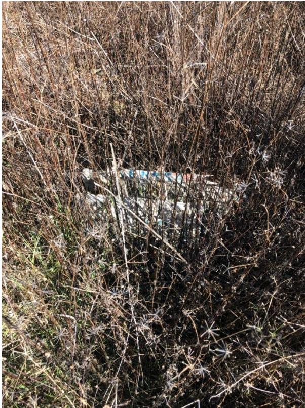
Figure 19 – View of heavily overgrown structure
