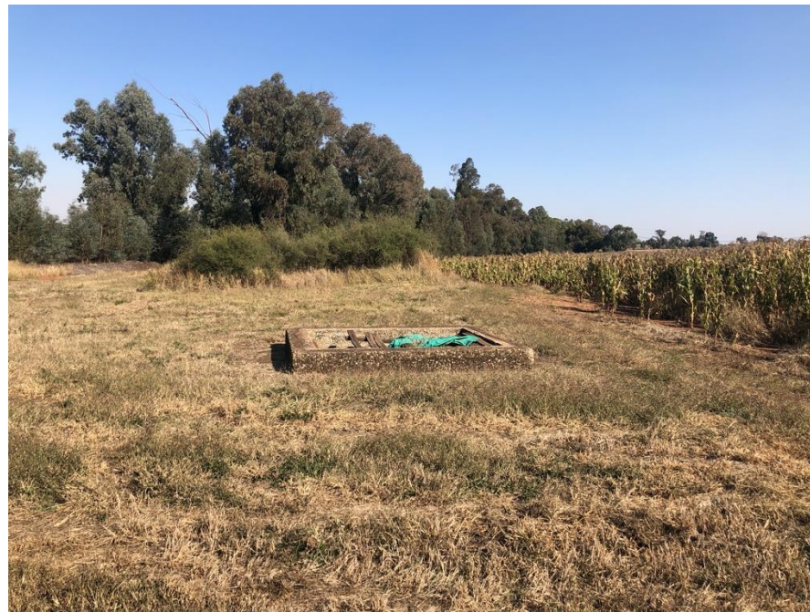
Figure 46 – View of the shaft collar of the vertical shaft at KF011
