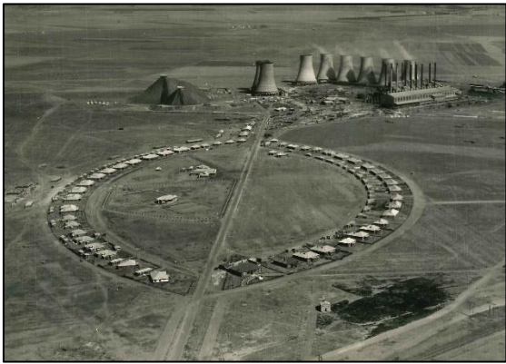
Figure 11 - Aerial view of Klip power station with the residential houses still under construction
