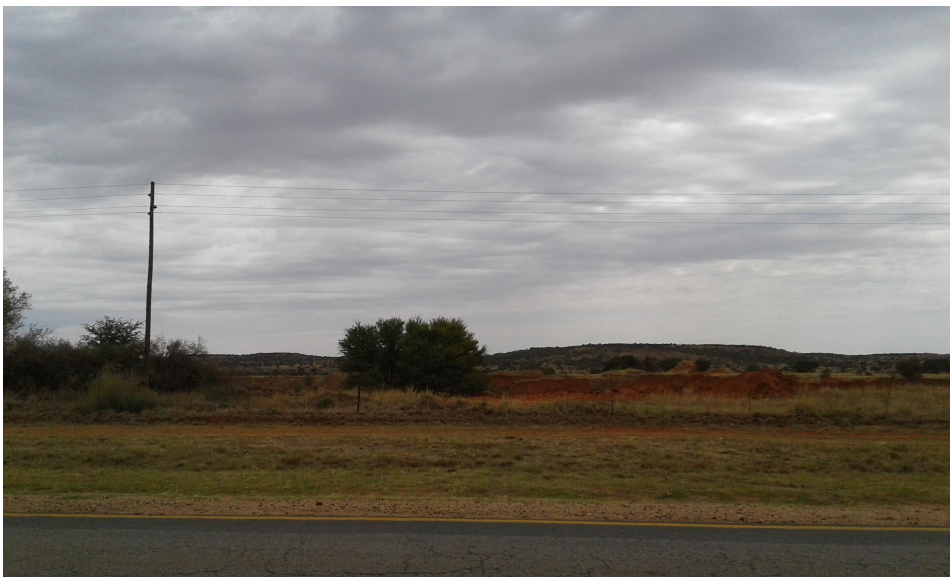
Figure 7: View of the road reserve on the eastern side of the R34.
