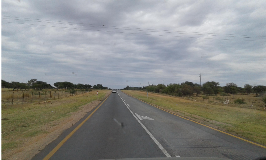
Figure 6: View along the R34. Note the large road reserve on both sides of the road.
