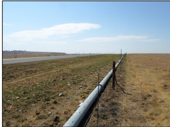
Figure 7 – General view of Area 3
