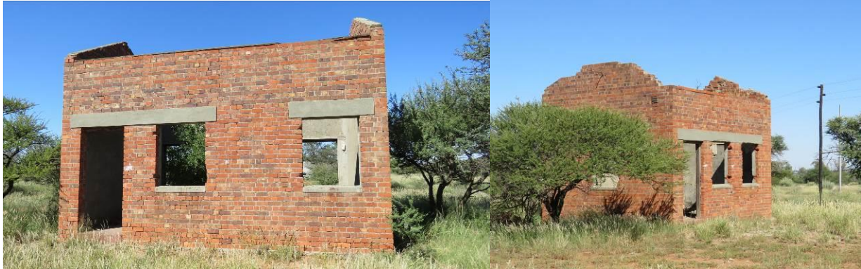
Figure 8: Pump infrastructure at 28.71370° 24.79055°
