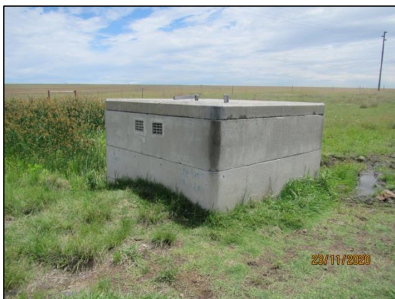
Figure 8 – Existing Pipeline/drain infrastructure identified throughout the site.
