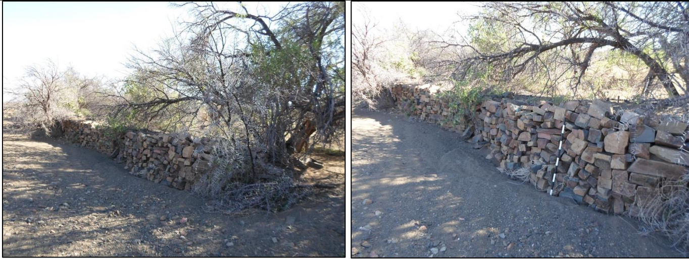
Figure 32: View of the packed stone wall or water break in the nearby stream at K012/4.
