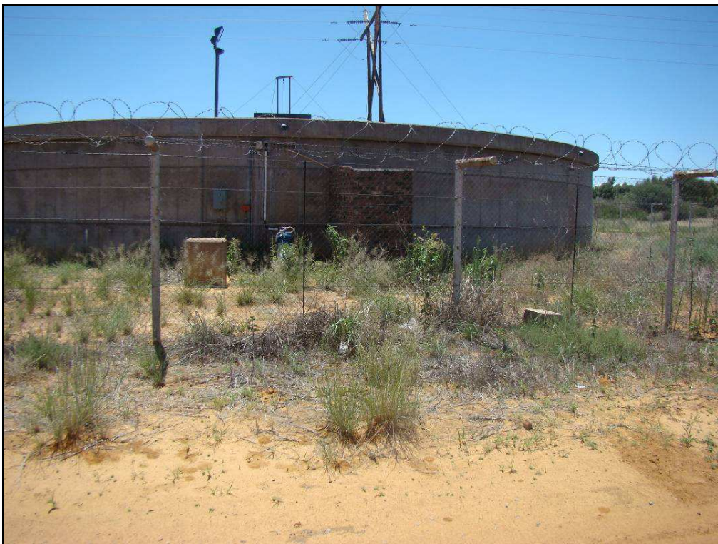
Fig.6 Water reservoir at Point D, Hotazel.
