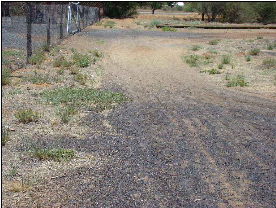
Fig.4 Eskom Sub-station at Hotazel new water pipeline route.
