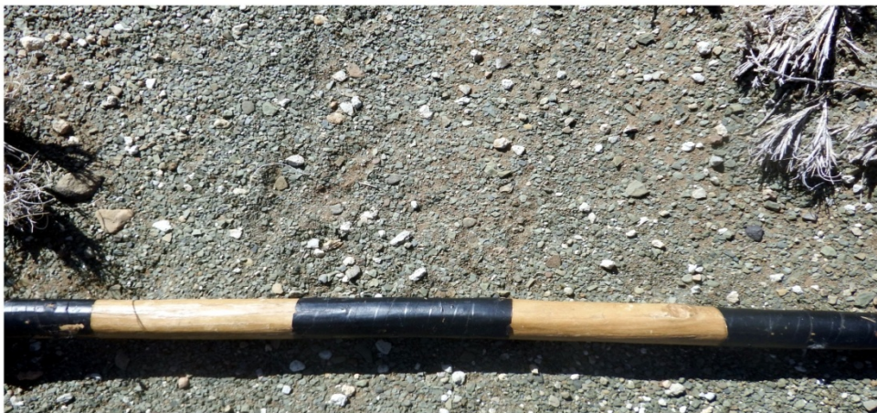
Figure 7. General view of the proposed pipeline route along the R361. The road has largely been constructed using locally available bedrock sediments (Ecca shales) for raw material (center and bottom). Scale 1 = 10 cm.
