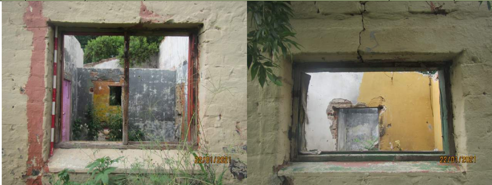
Figure 22 – Alternate views of structure at WK002
