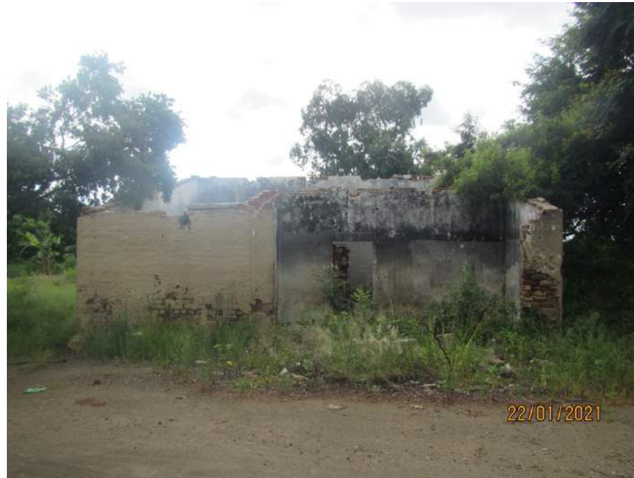
Figure 21 - View of the western facing wall.
