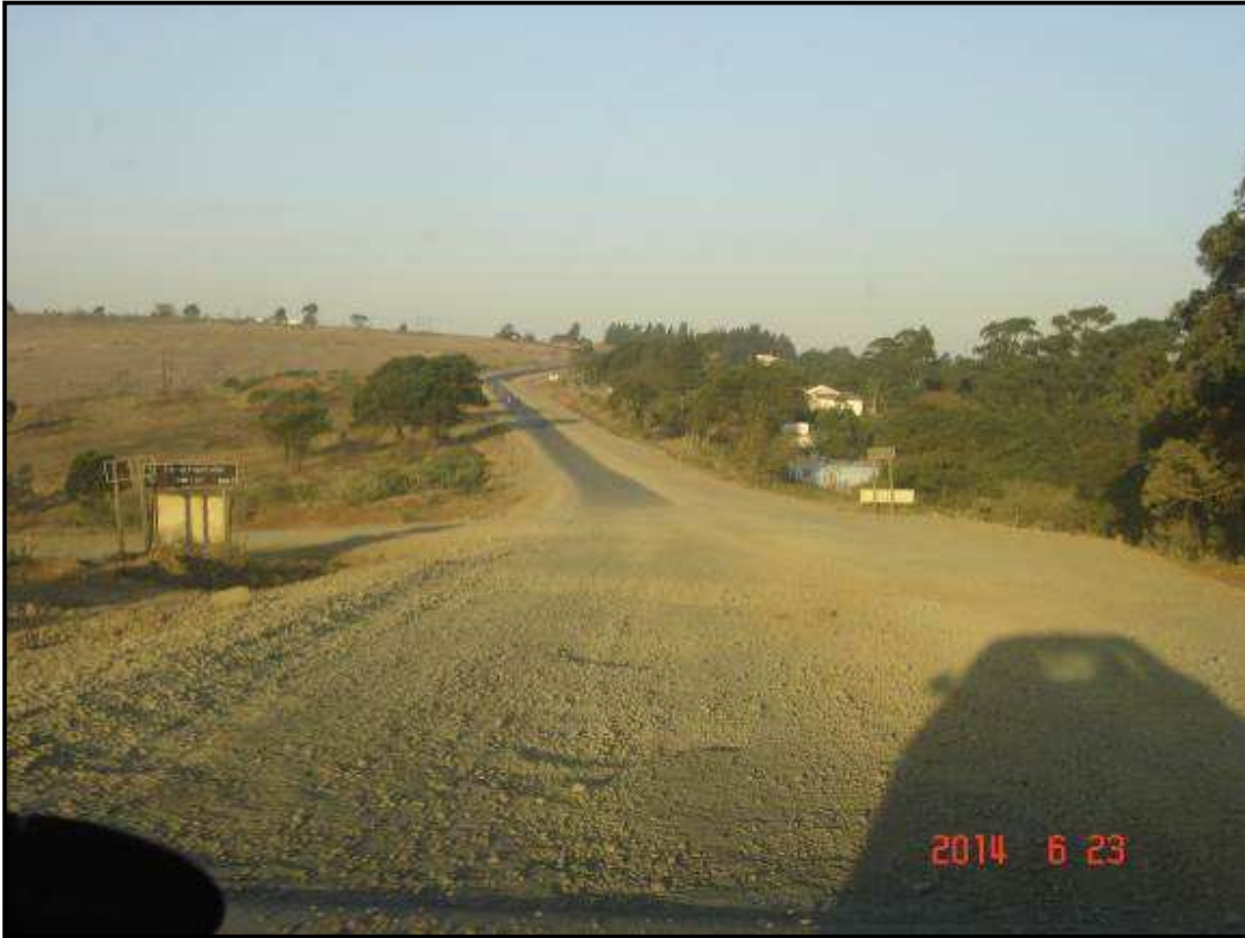
Plate 1: Road Section to be upgraded (visibility fair)
