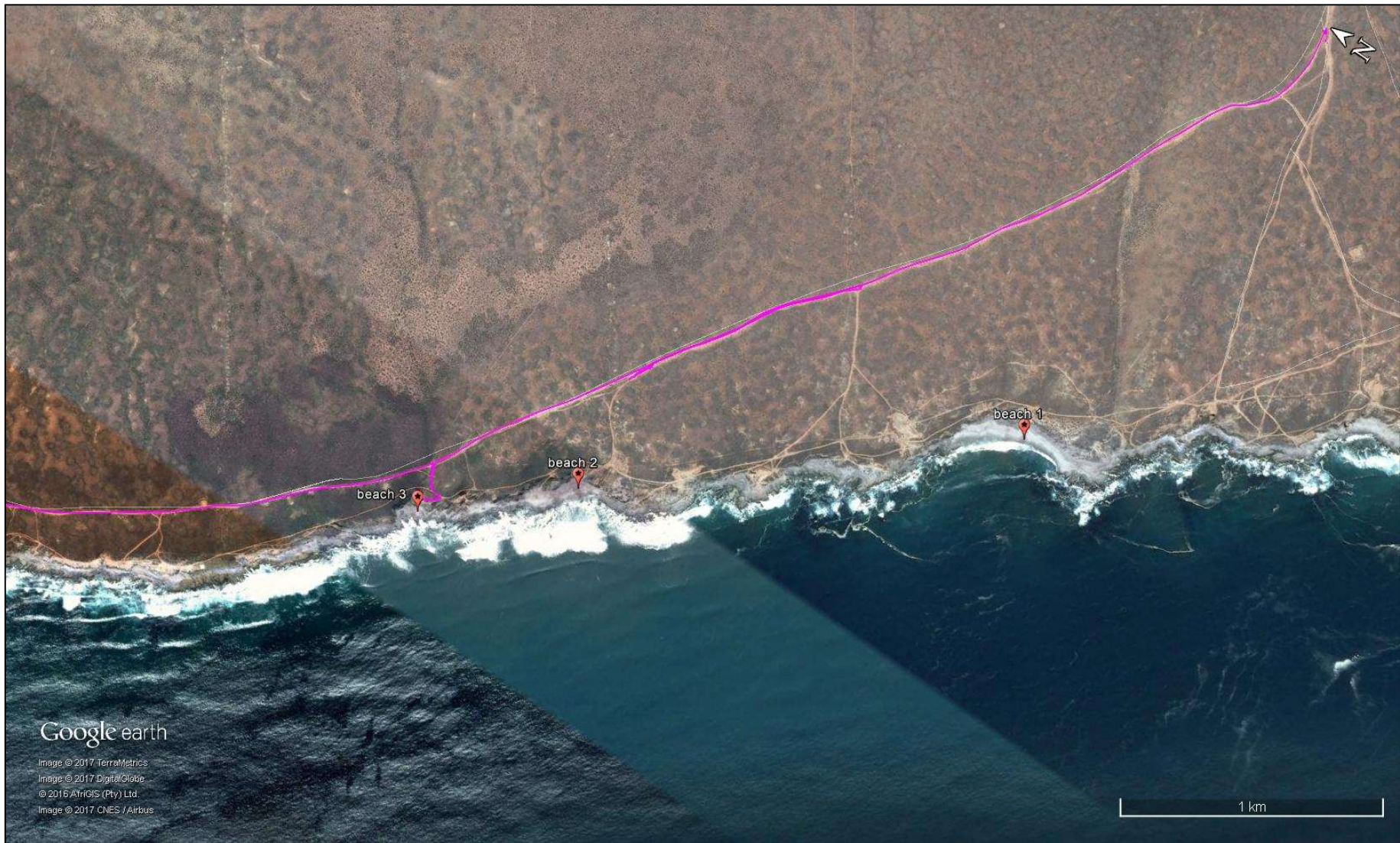
Figure 3-2: Assessment of beach mining expansion and access roads, track paths (magenta lines)
